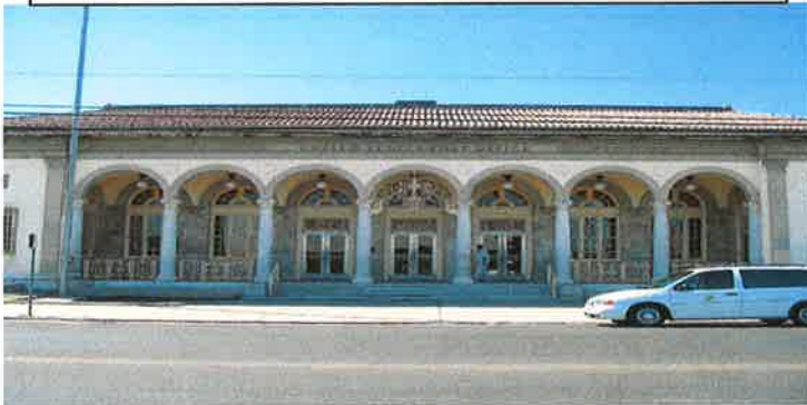
Design Build Historic Restoration
