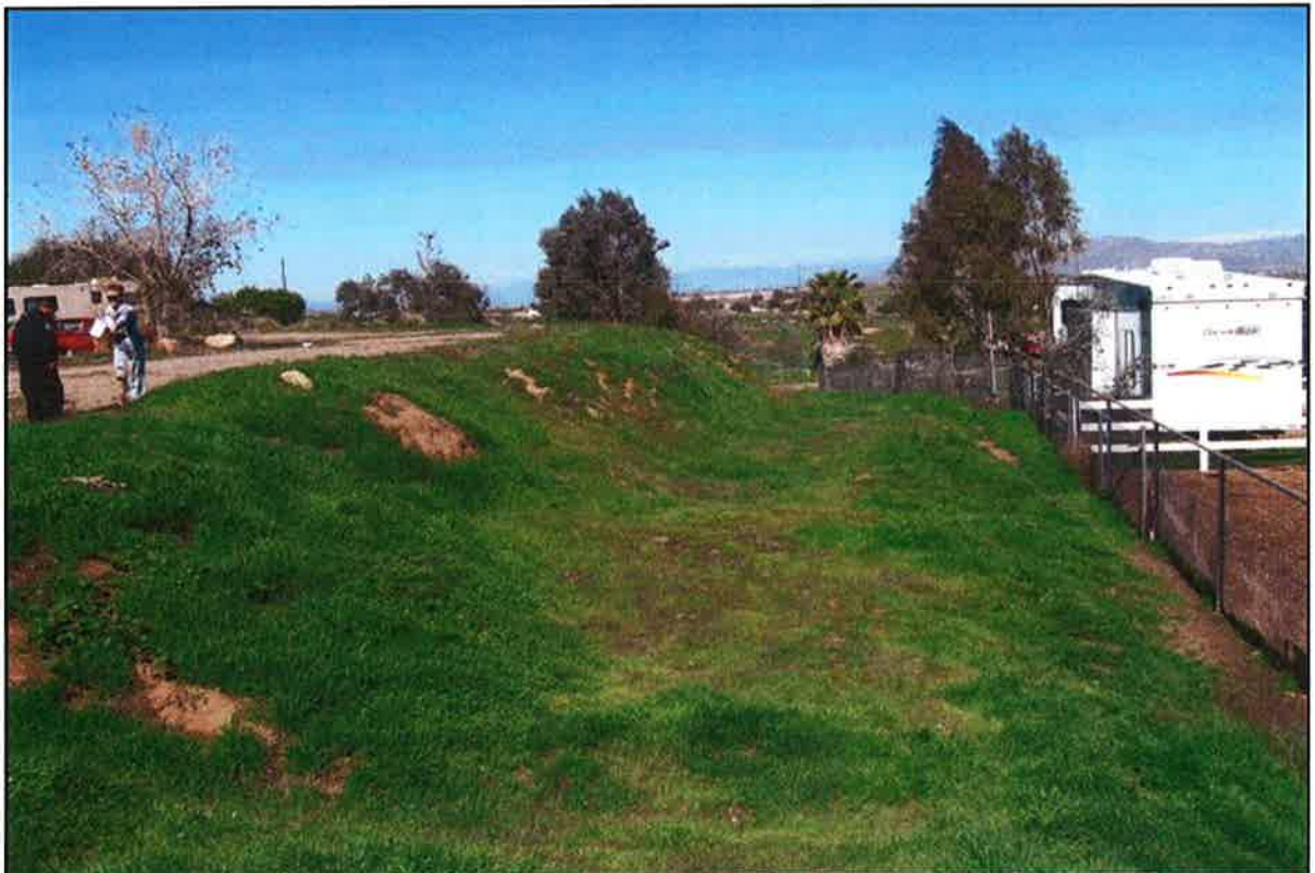
R Welch PHOTO # NOTES: Looking North on the East prop line
