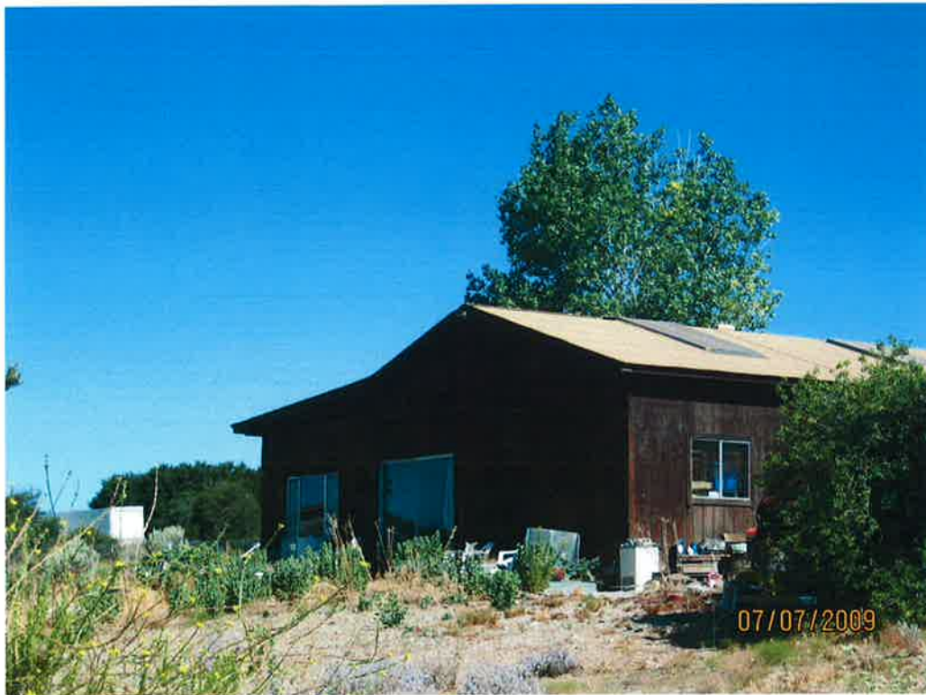
PHOTO # 3 NOTES: from the Road right-of-was EOS & AR
