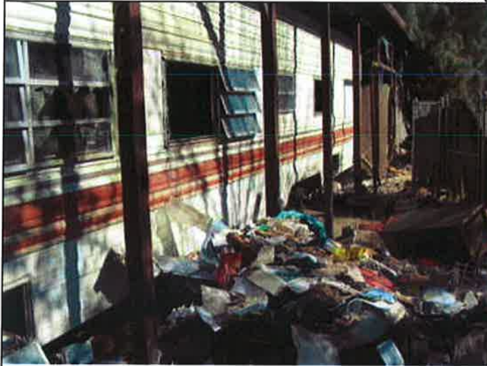
Accumulation of Rubbish and Excessive outside Storage
