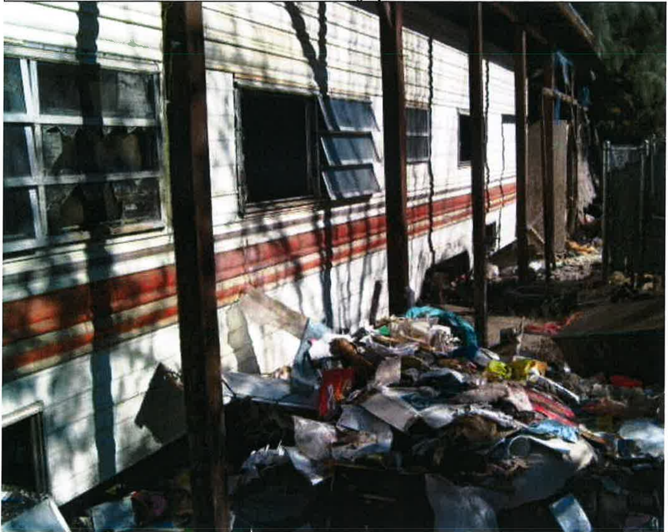
Accumulation of Rubbish and Excessive outside Storage - 07/17/2010
