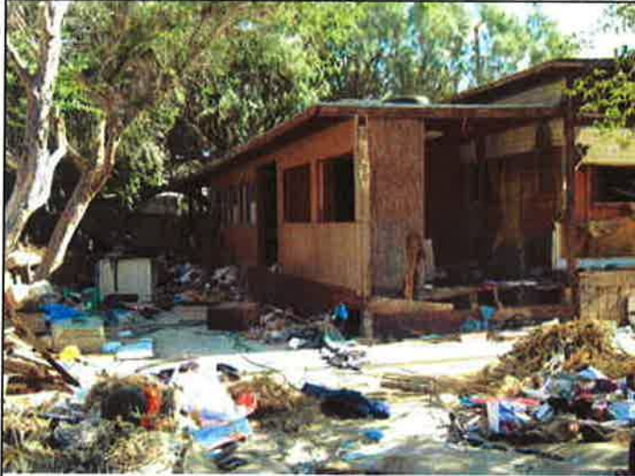
Accumulation of Rubbish
