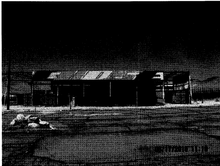
061710, CV1003317 - Substandard Structure / T Cervantes - 06/17/2010
