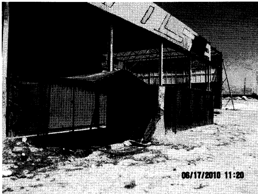
Notice of Defects #11 - Members of Ceilings, roofs, ceiling and roof supports or other horizontal members which sag, split, or buckle due to defective material or deterioration. #14 - General Dilapidation or improper maintenance. #17 - Public and attractive nuisance - abandoned/vacant / T Cervantes - 06/17/2010
