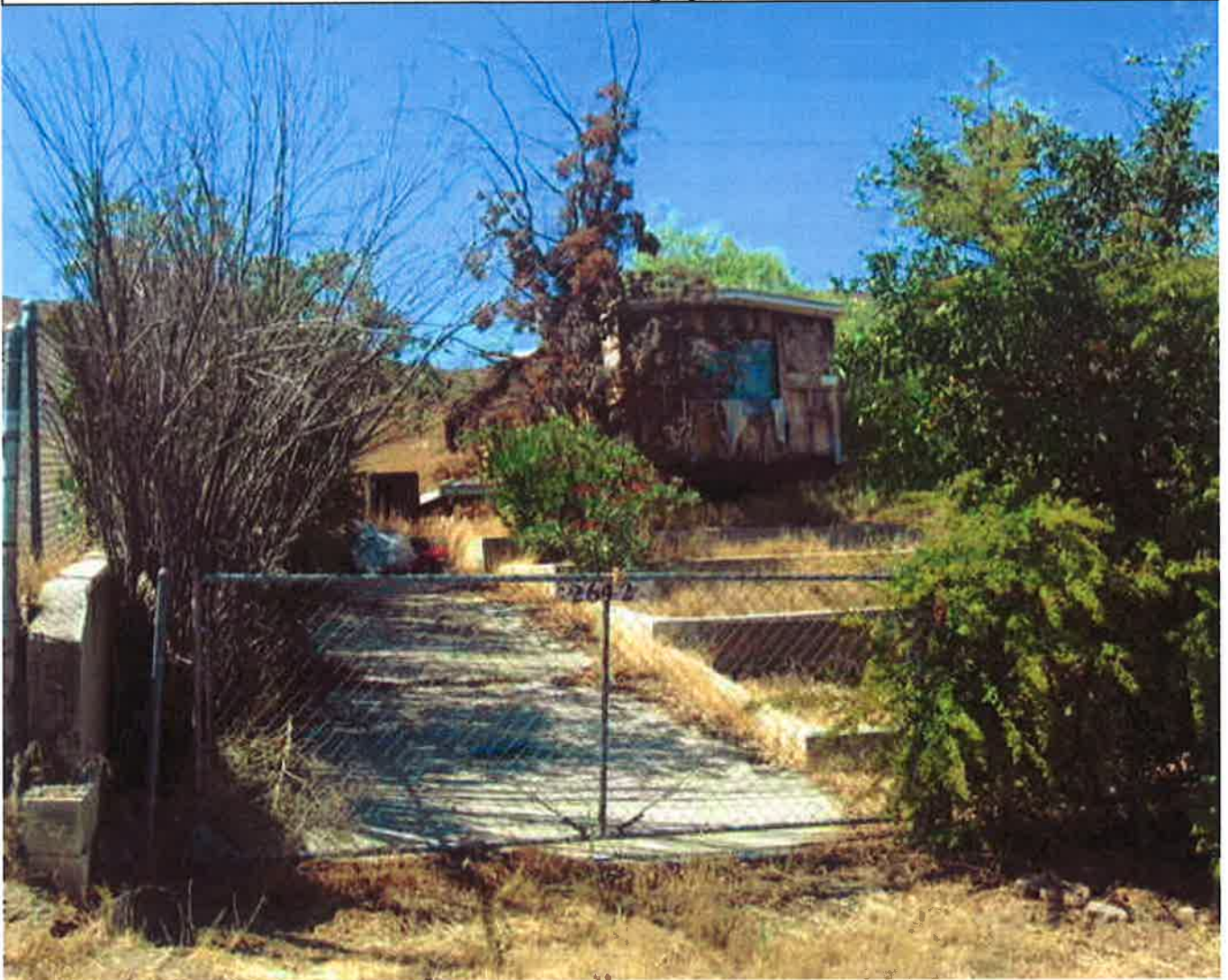
E. Torres; violations remain, no improvements - 08/11/2010
