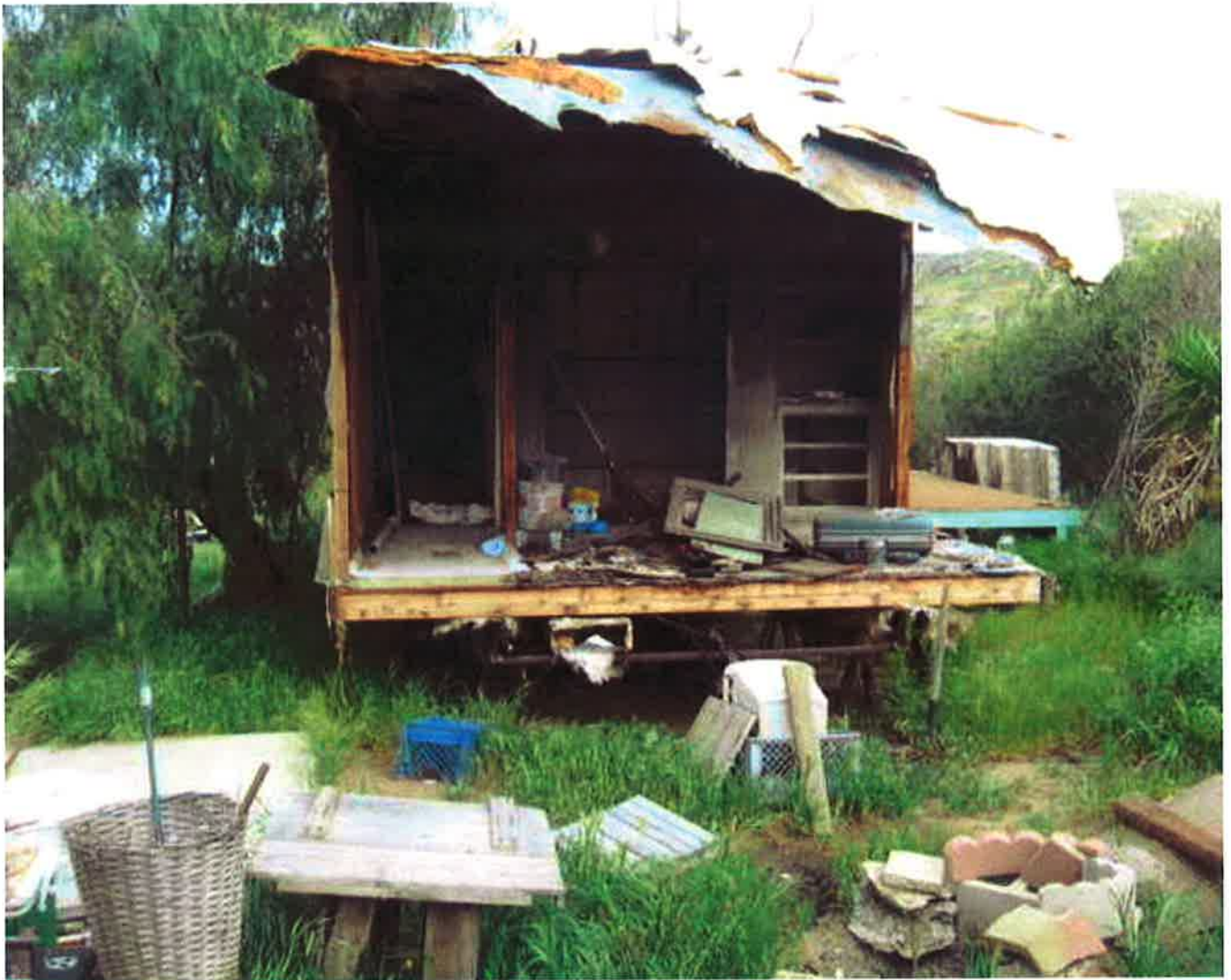
E. Torres; defects-10, 12, 13, 14, 16, 17, 19 - 03/31/2010
