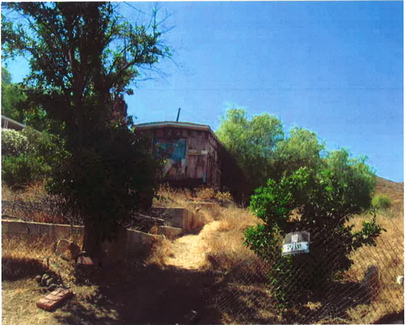
E. Torres; violations remain, no improvements - 08/11/2010
