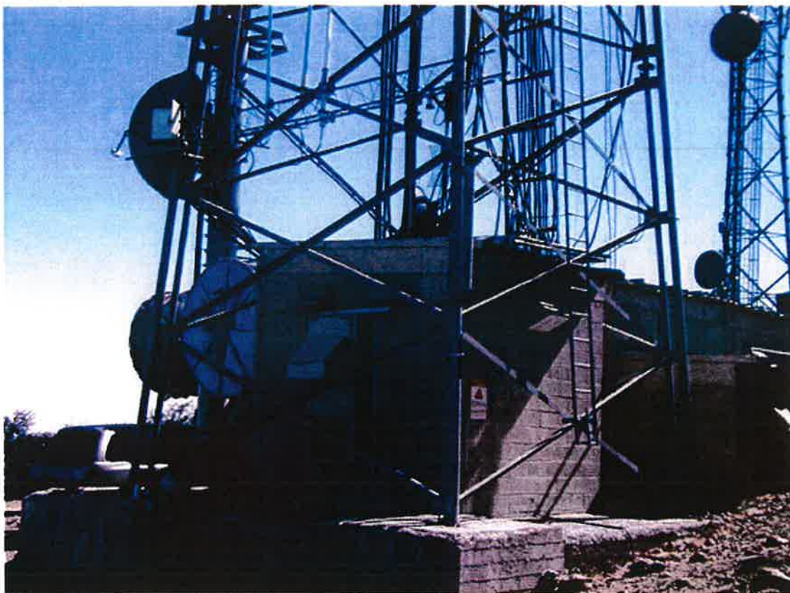
Small Bldg and tower base from west
