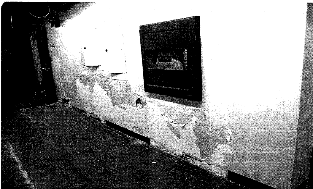
Picture 16 – Water-damaged interior partition
