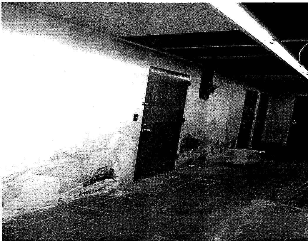
Picture 17 – Water-damaged interior partition
