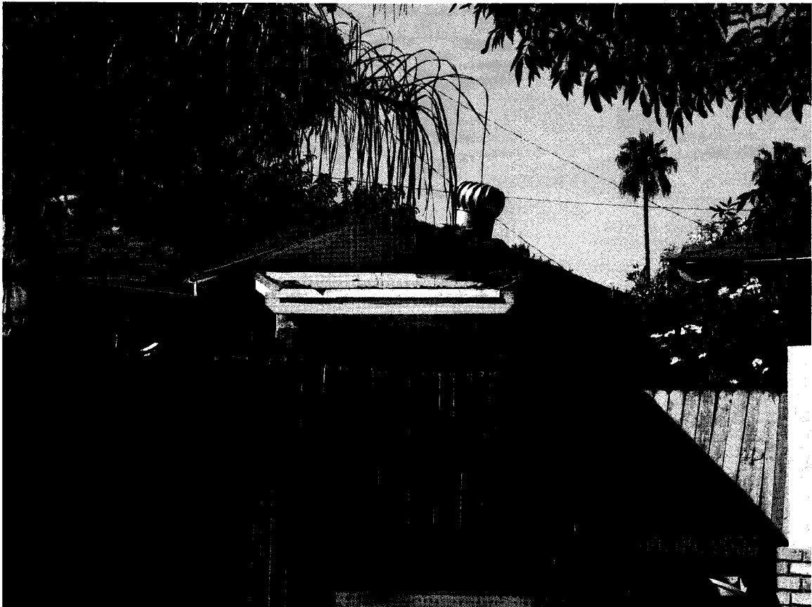
PHOTO #4 CWP & ENCROACHMENT
