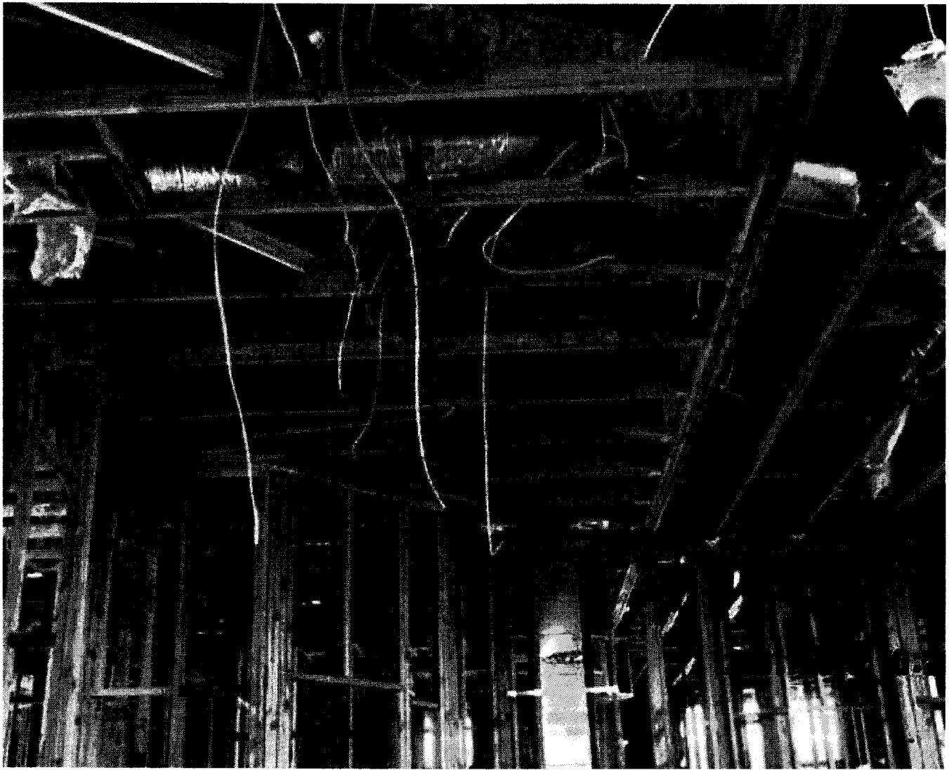
Photo #8 - defect 5 and 7 - 12/01/2010
