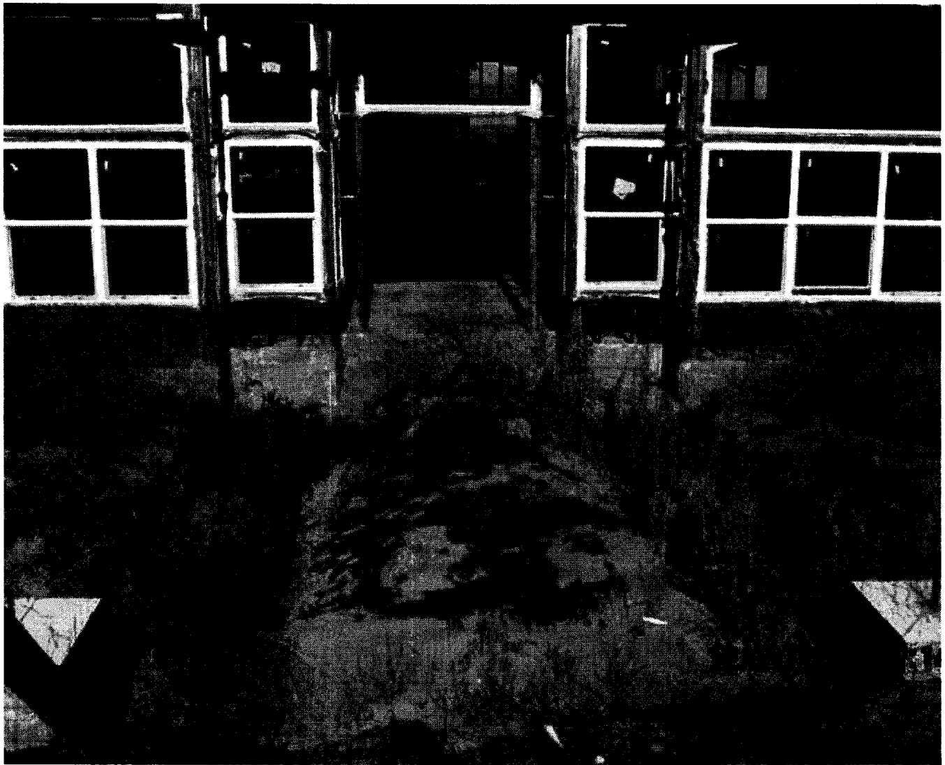
Photo #3 - entry missing door - defect #13 - 12/01/2010
