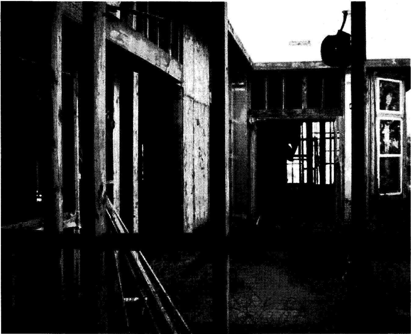
Photo #6 - defects 12 and 13 - 12/01/2010
