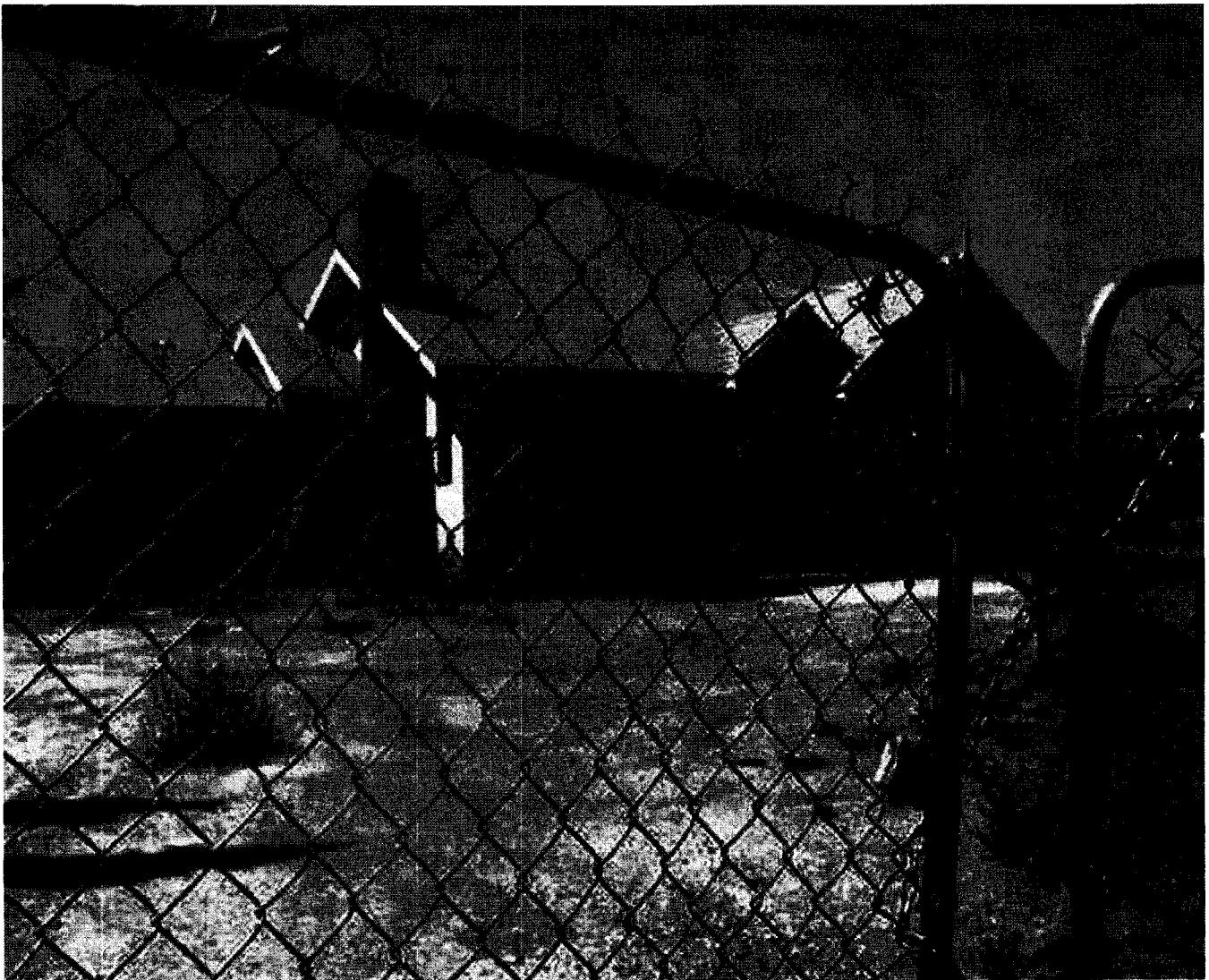
Structure remains substandard-JMorris 7/15/10 - 07/15/2010
