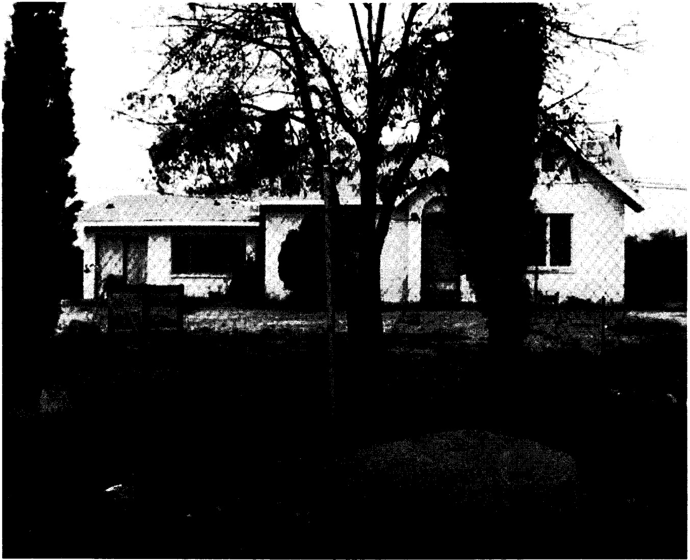
Structure remains substandard-JMorris 12/21/10 - 12/21/2010
