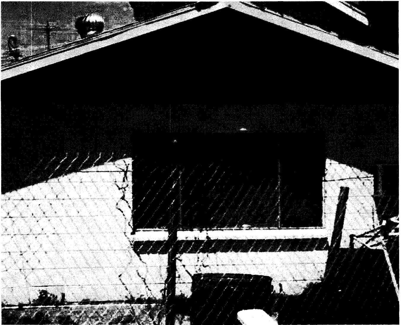
Structure remains in substandard condition-JMorris 5/25/10 - 05/25/2010
