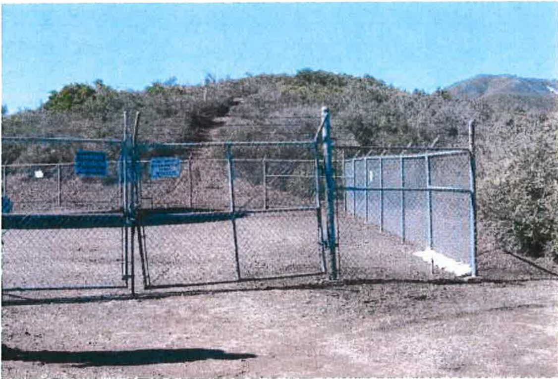
Facility 2 – Riverside County (Proposed Development Area is Located Within the Fence-line)
