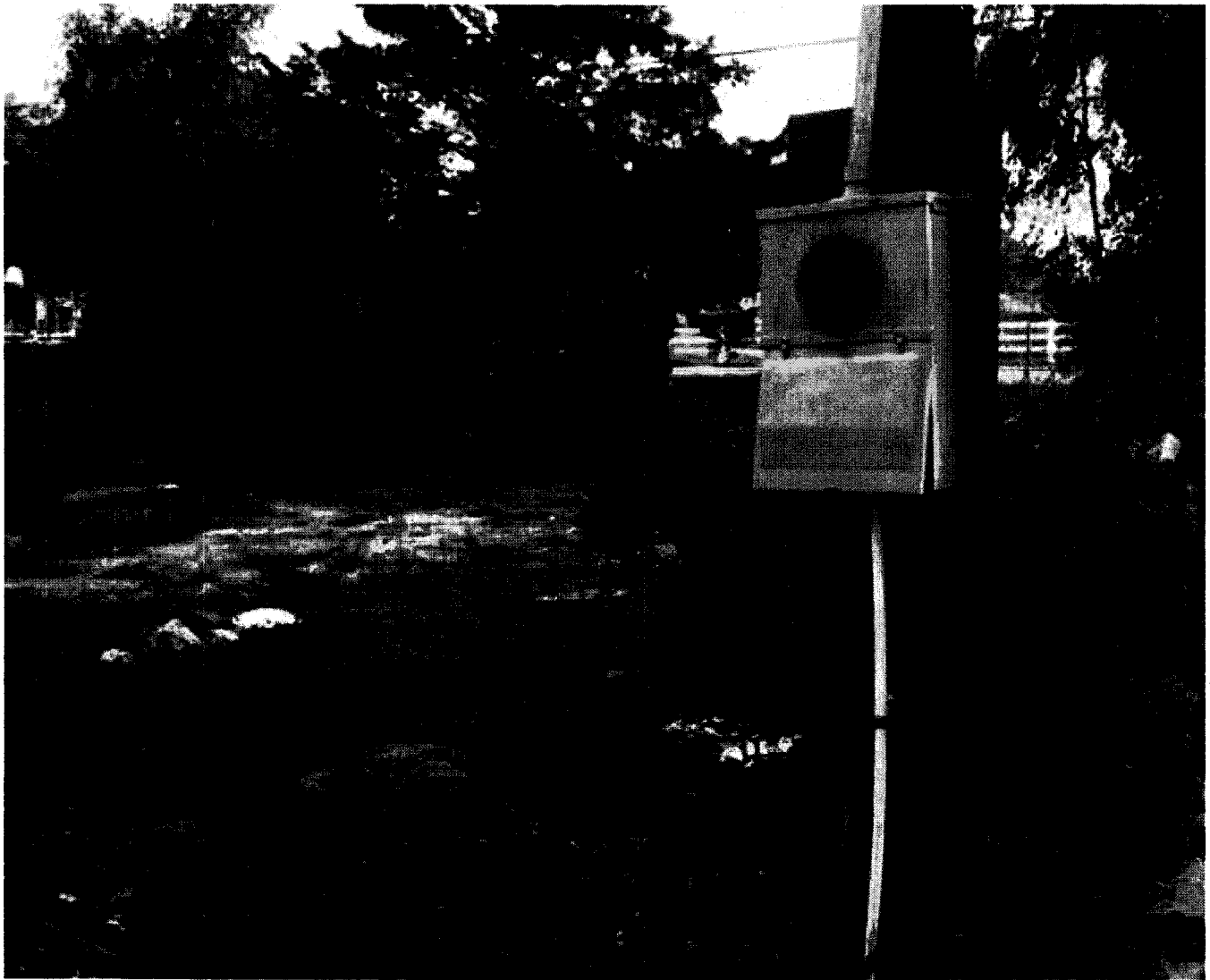
photo #3 - electrical meter removed - 01/05/2011
