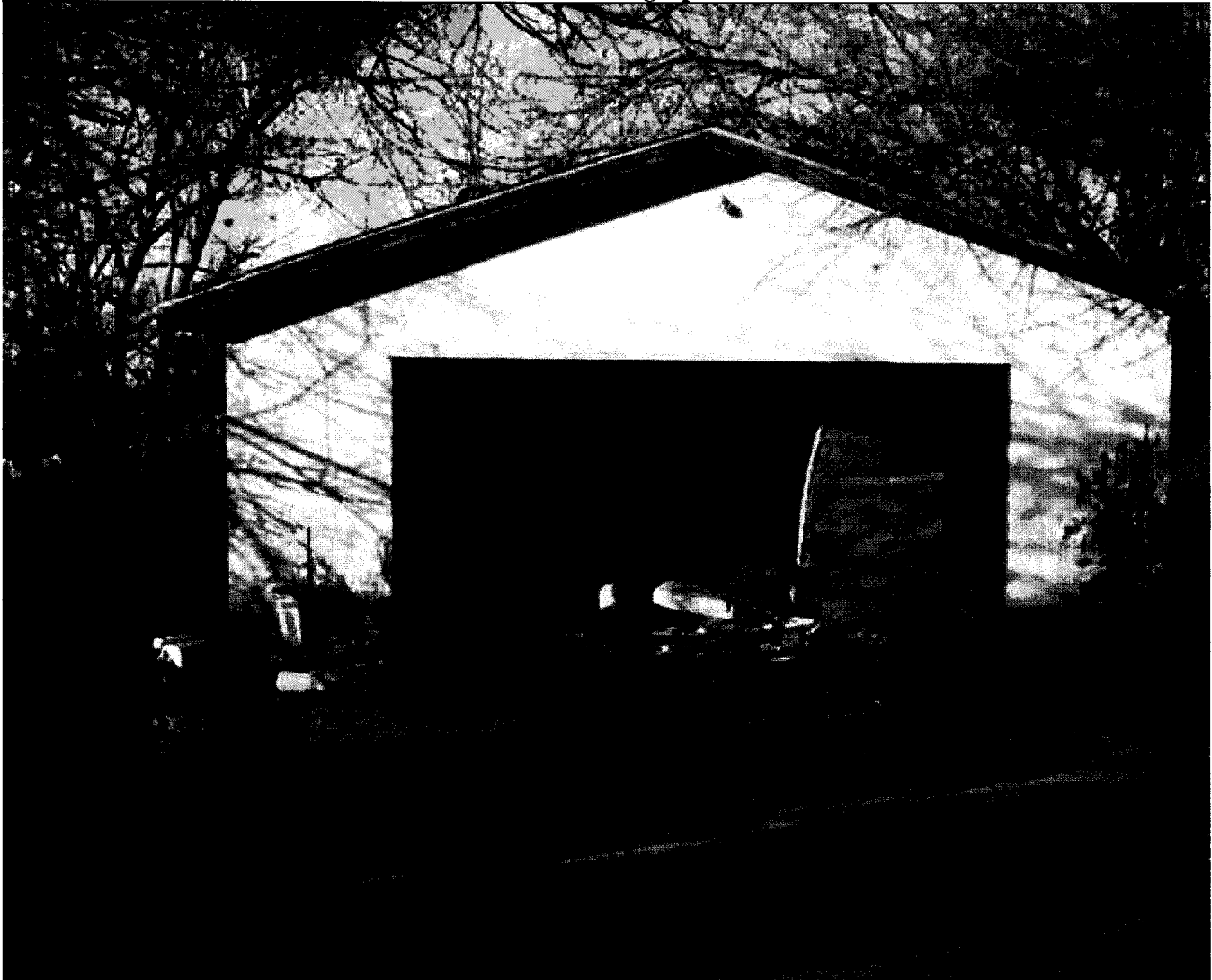
Photo #1 - substandard garage and rubbish - 02/01/2011
