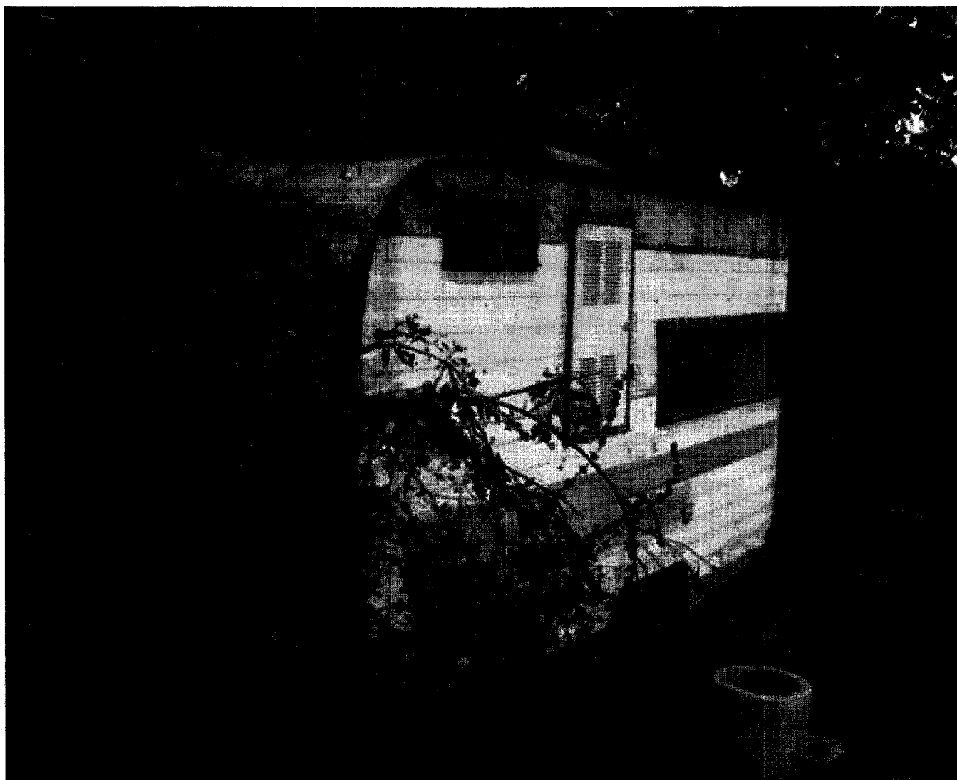
PIC#8 SSTT DEFECT#14&17 J.Kirchoff - 09/08/2010
