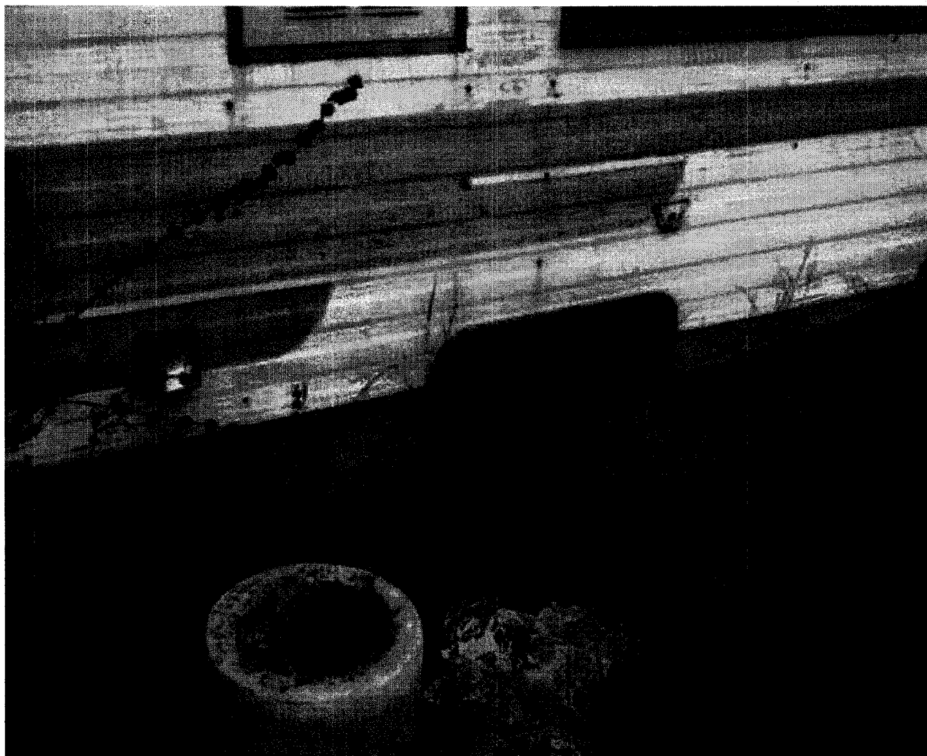
PIC#9 DEFECT#14 J.Kirchoff - 09/08/2010
