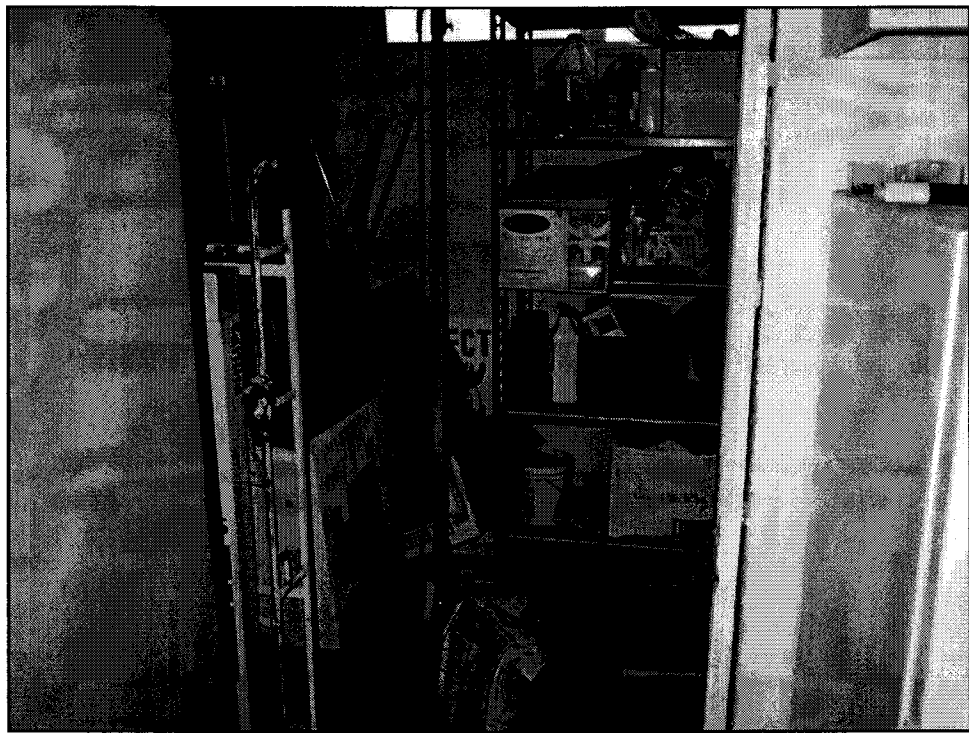
Photograph 20 – View of the cleaning storage area within the kitchen area of the Moose Lodge.
