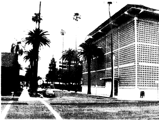
Photo 3: Staging area on 11th Street
