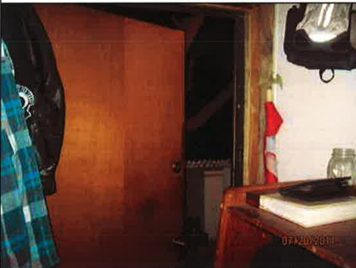
North exit door located in room addition.
