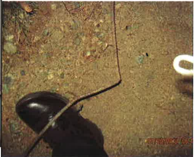
Johnston, Defect #6 - grounding wire from svcs panel deteriorated
