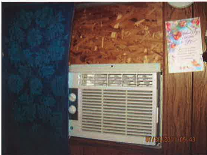
Johnston, Defect #15 - Window blocked water cooler installed at window
