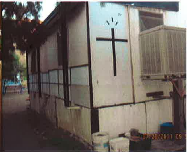
Johnston, Defect #19 - Substandard/illegal roof addition to mobile
