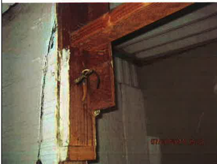
Exterior exposed wood framing.jpg
