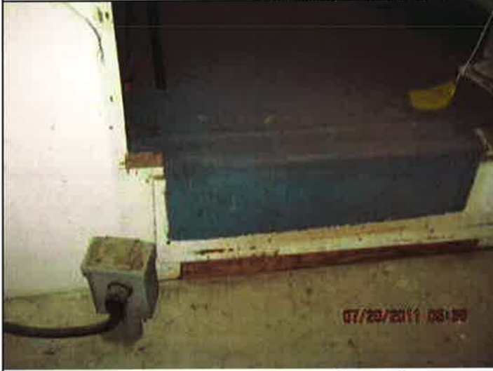
16in. step in bunk room-porch area.jpg
