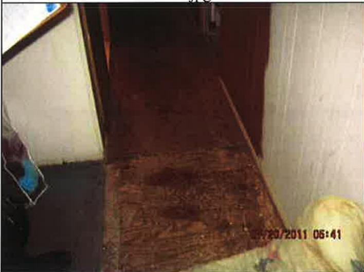
exposed plywood floor.jpg
