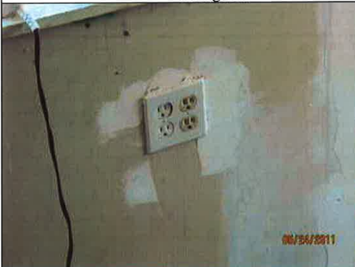
Electrical covered as requested. JHeagstedt
