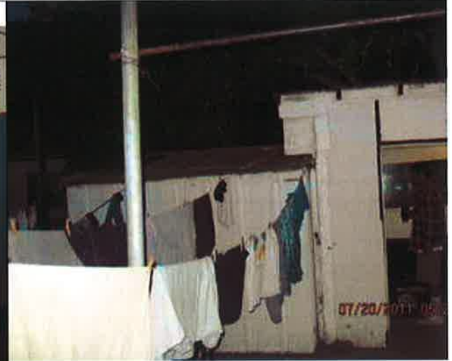
Enclosed carport with attached metal shed addition.jpg
