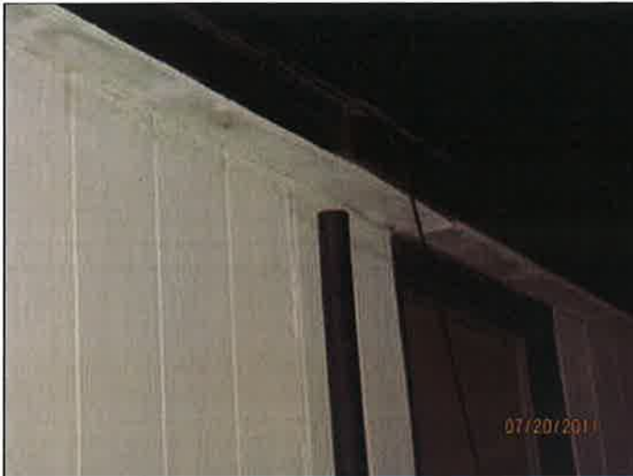
vent pipe below roof line of mobile/ D.Parra
