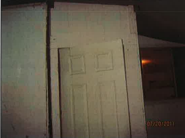
exterior of unpermitted bathroom/D.Parra
