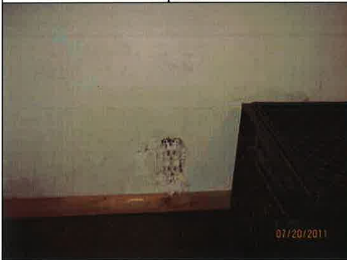
electrical outlet without cover/D.Parra
