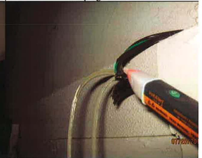
spliced electrical to air conditioner energized/D.P
