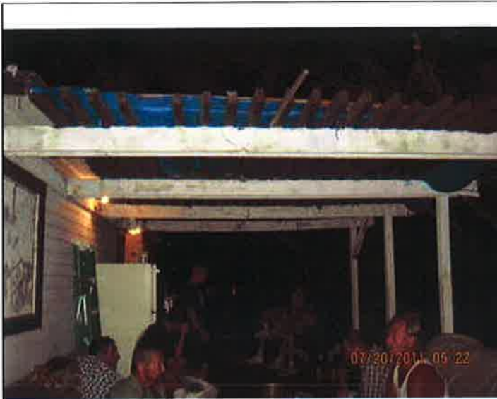
lattice patio cover attached to structure
