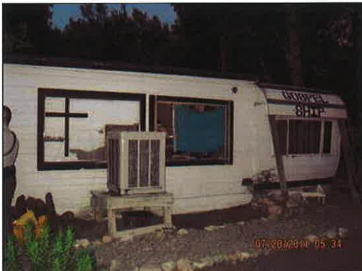
enclosed patio and addition to mobile. M. Villanueva
