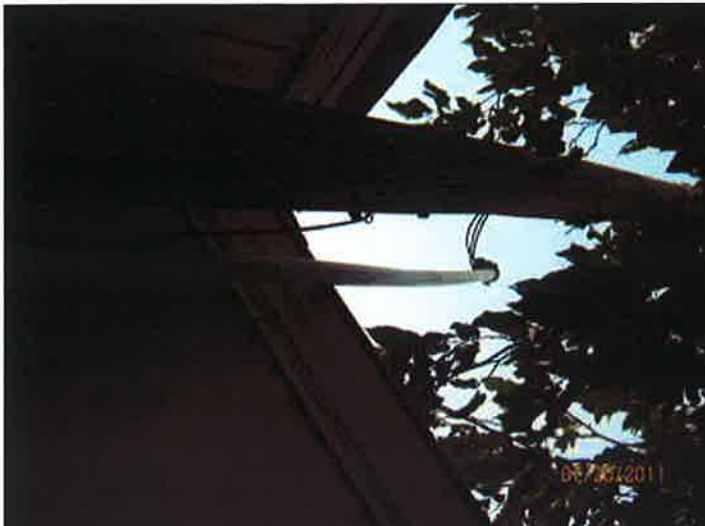
CForrey / 07/20/11 Defect # 6 main power supply not secured to power pole
