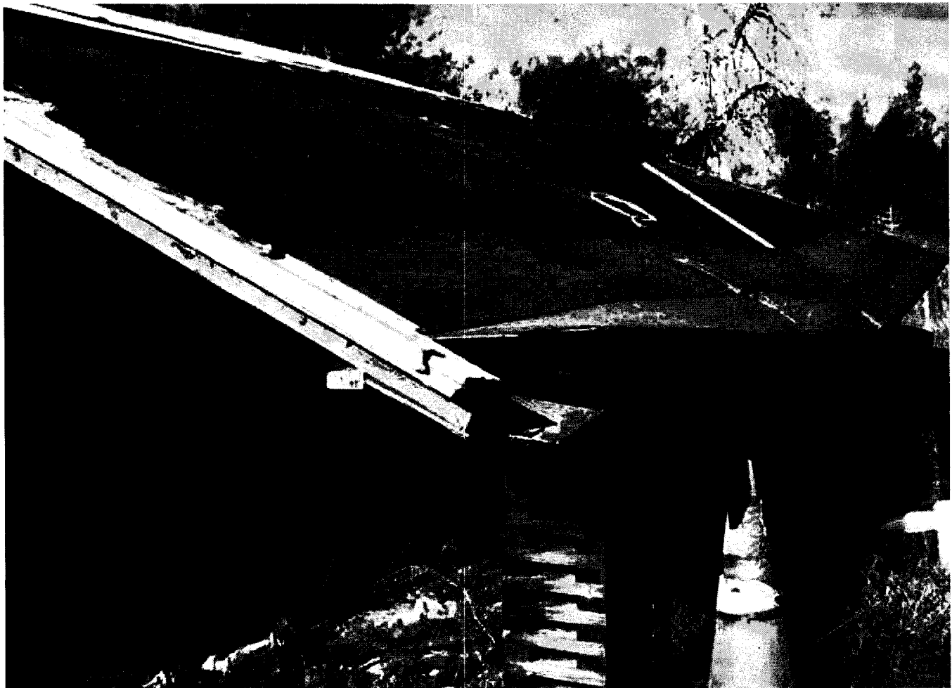
Taken by CEO Lyon - The lean-to has no solid support, is dilapidated, roofing material is gone and it is apart. NOD#10,11,13,14,17 - 02/16/2010
