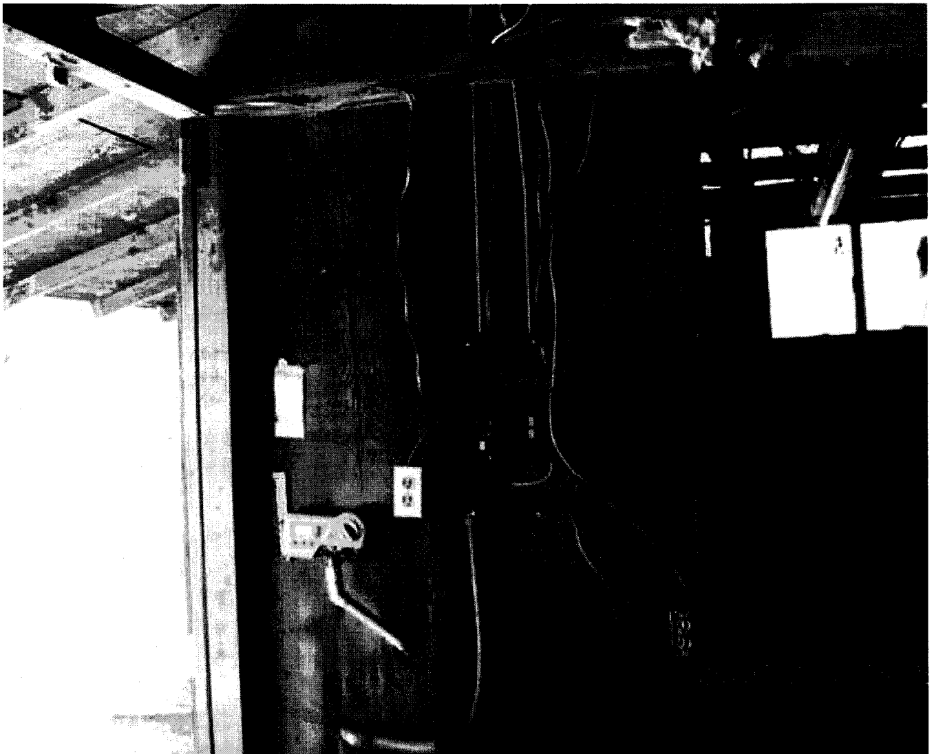
Photo #7 - Defect 6 RW_ substandard and exposed electrical - 05/04/2010
