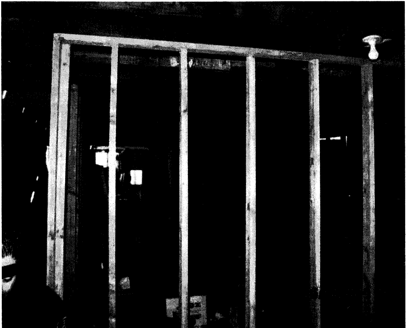
Photo #4 - Defect 10 RW_ new framing inside struction - 05/04/2010
