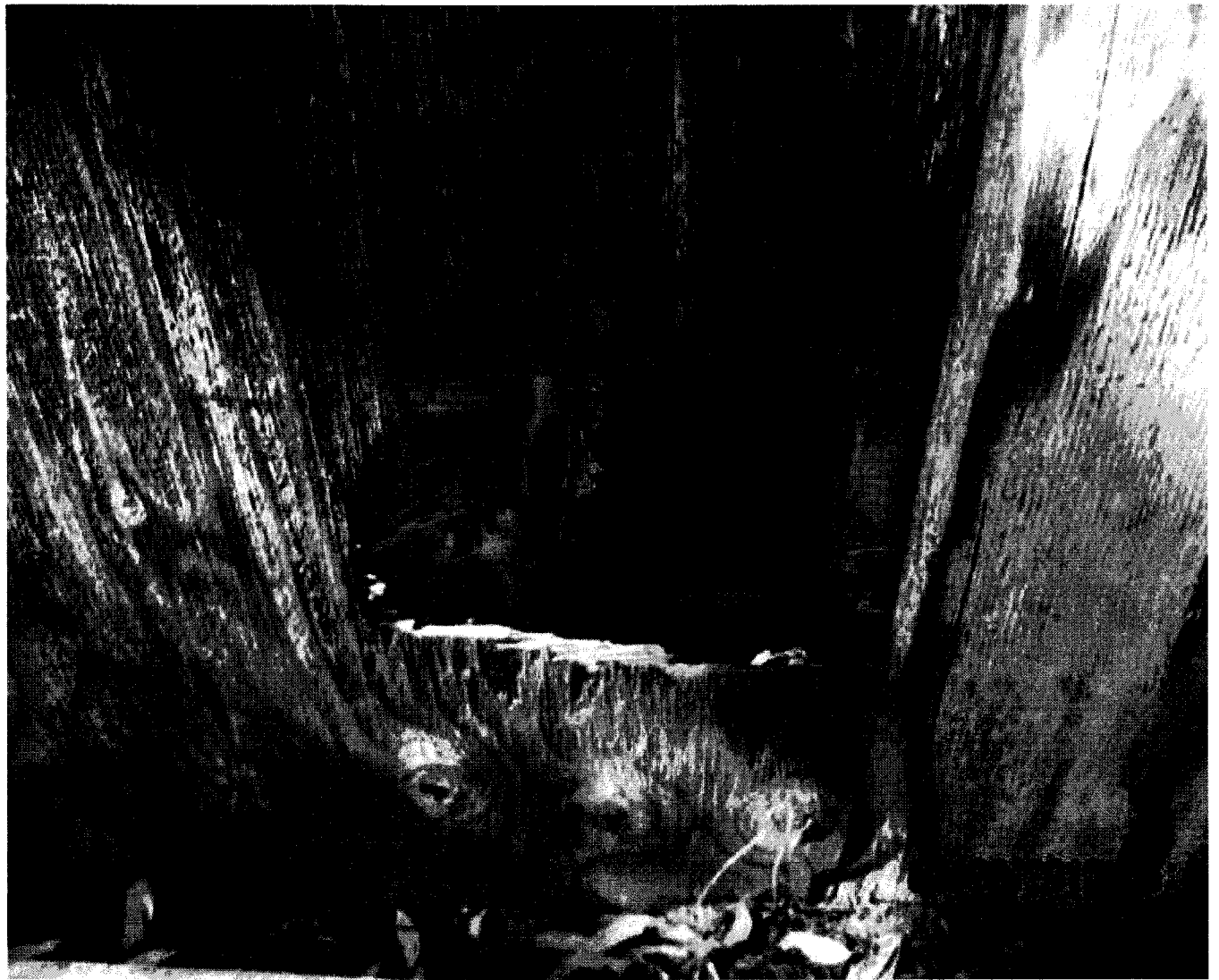
Photo #16 - Defect 14 RW_holes in siding - 05/04/2010
