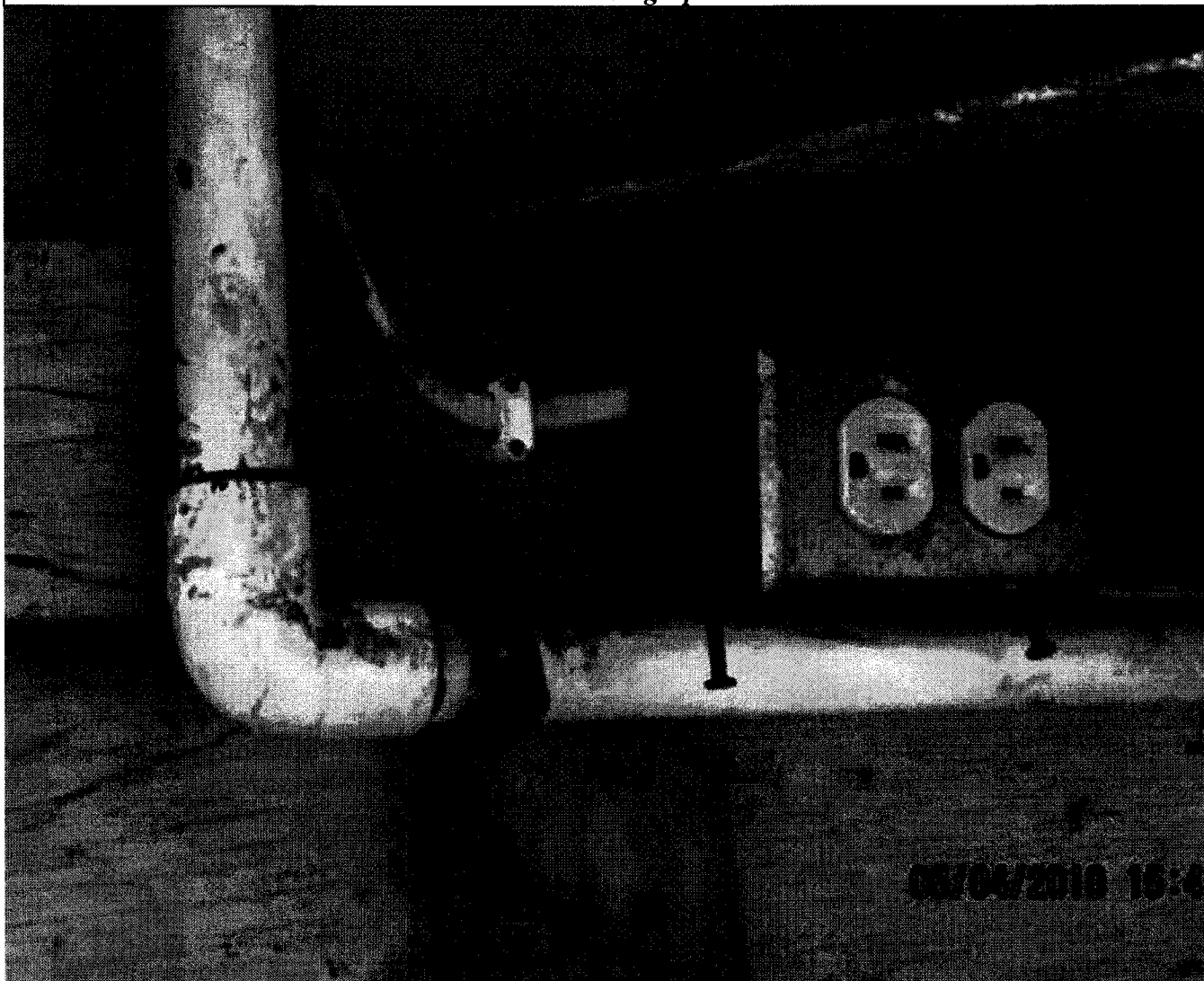
Photo #1 - Defect 6 RW_ exposed electrical, and added plumbing - 05/04/2010
