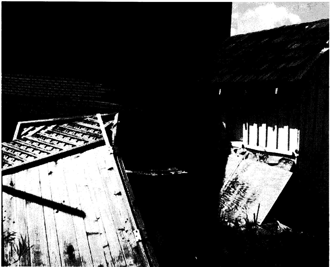
Substandard shed #1. Defects 10, 11 & 14. Lpadilla 3/22/2011 - 03/23/2011
