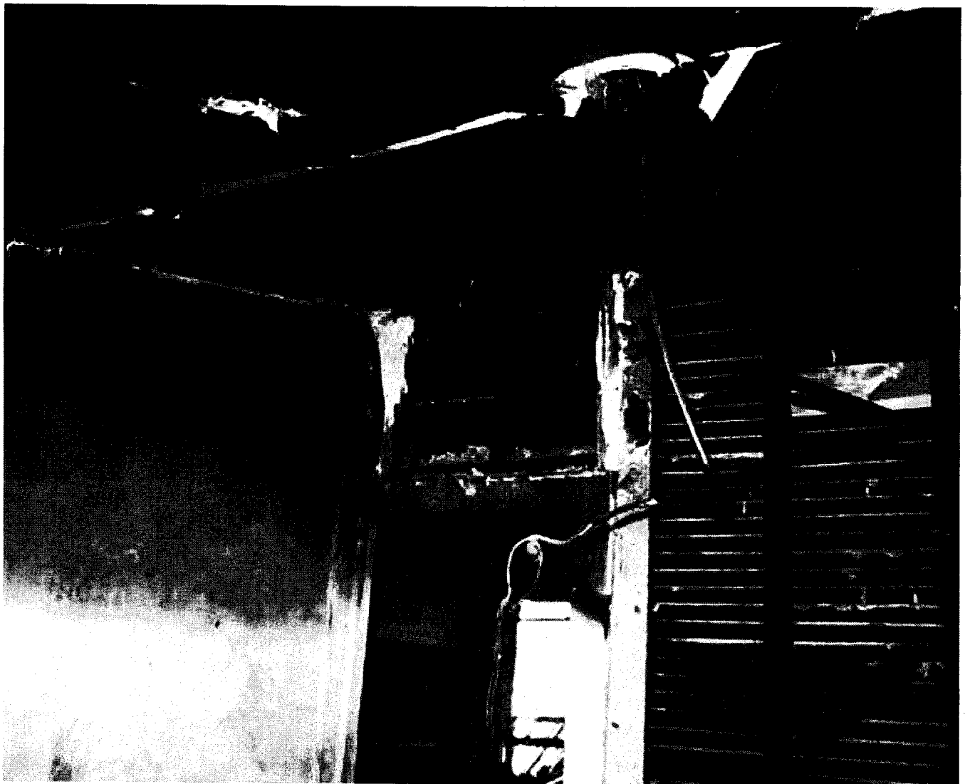
Fire damage roof in kitchen. defect 6,11, 14 & 16. Lpadilla 3/22/2011 - 03/23/2011
