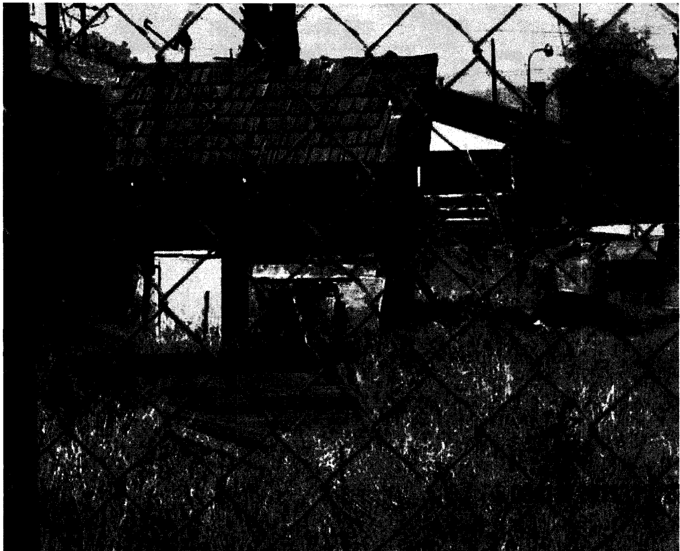
Substandard shed #2. Lpadilla 5/13/2011 - 05/13/2011
