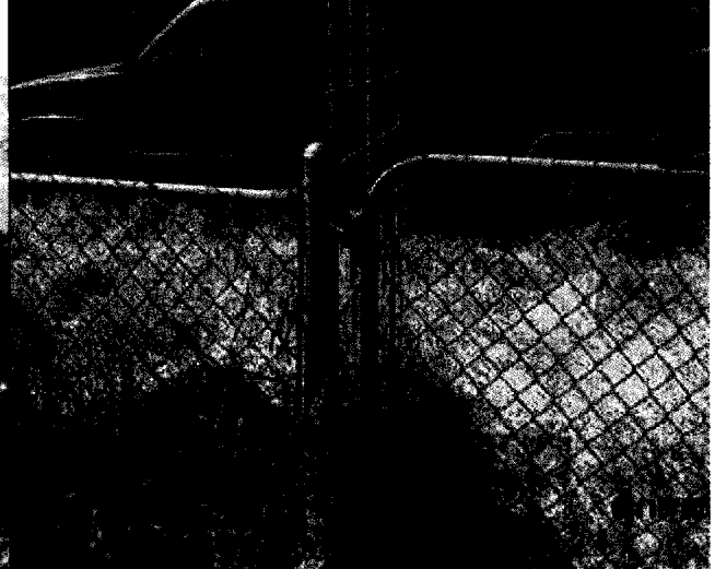
M Sanders 061510 - open walk through gate, no postings to prohibit entry
