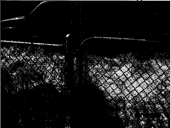
M Sanders 061510 - unlocked walk through gate, no signs prohibiting entry
