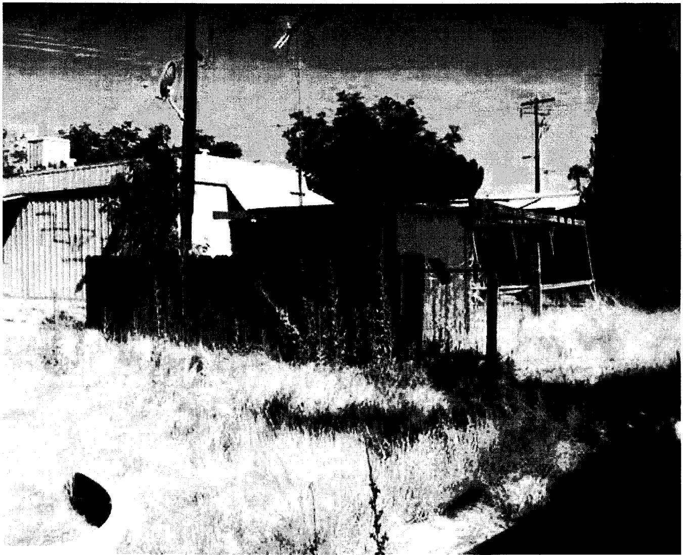
Torres; accessory structure/arbor-defects 10, 11, 14, 17, 19 - 06/25/2010
