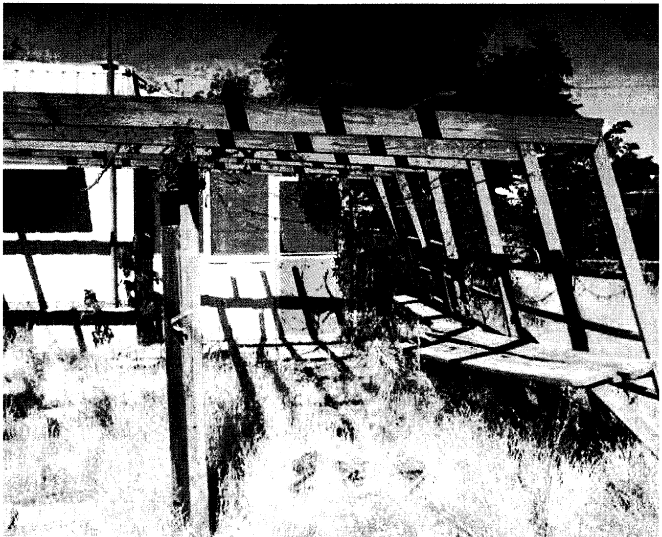
E. Torres; arbor listing to one side-defects 10, 11, 14, 17, 19 - 06/25/2010
