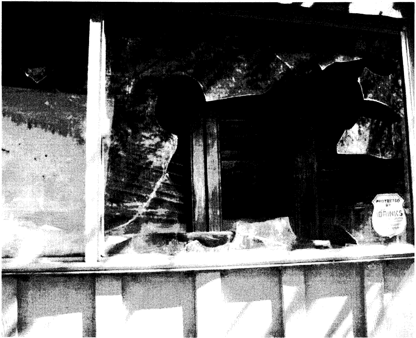
E. Torres; broken window-defects 12, 13, 14, 17 - 06/25/2010
