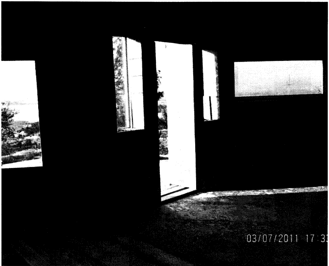
Photo #13 - Defect 13 - no door - 03/07/2011
