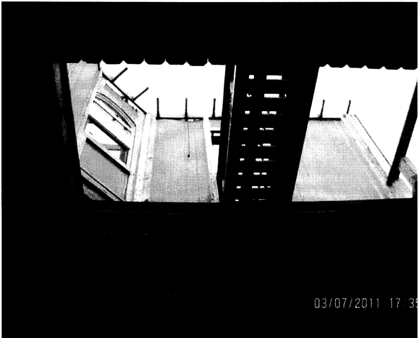
Photo #15 - Defect 11 - no roof or ceiling - 03/07/2011
