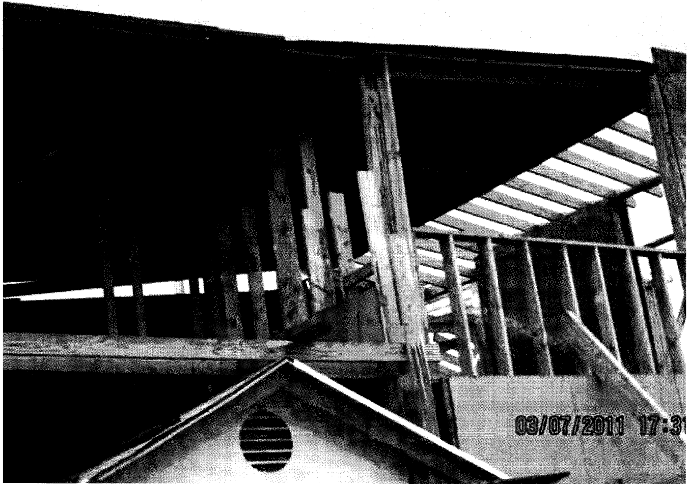
Photo #2 - Defects 12 and 13 - 03/07/2011
