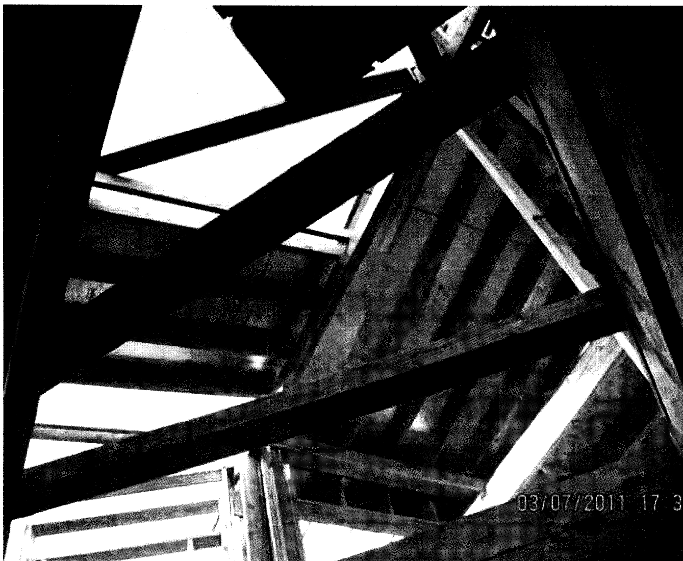
Photo #11 - Defects 11,12 and 13 - 03/07/2011
