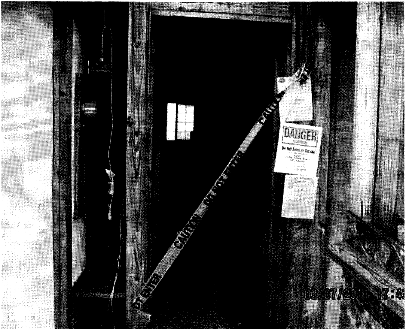
Photo #19 - Defect 17, open sliding door - public nuisance/posting - 03/07/2011
