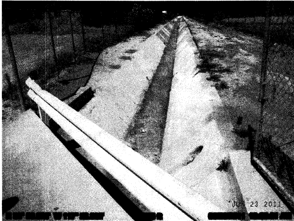
Photo #1: View of Lime Street Channel at the outlet location.
