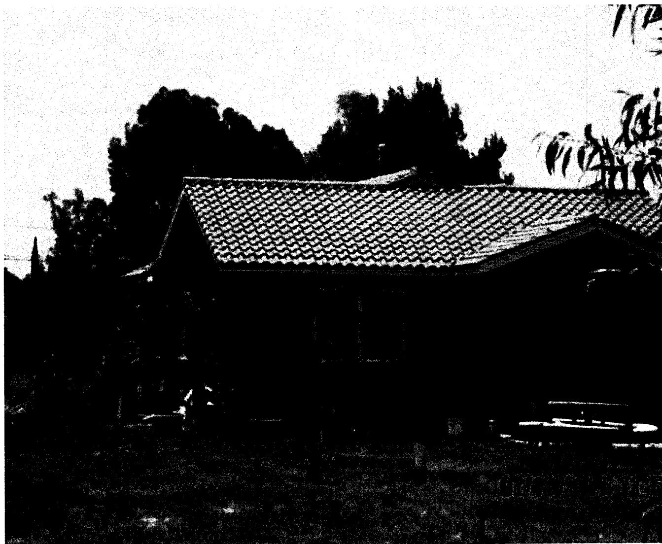
from r/o/w, no exterior siding to the substandard structure; by SCervantes - 07/13/2011
