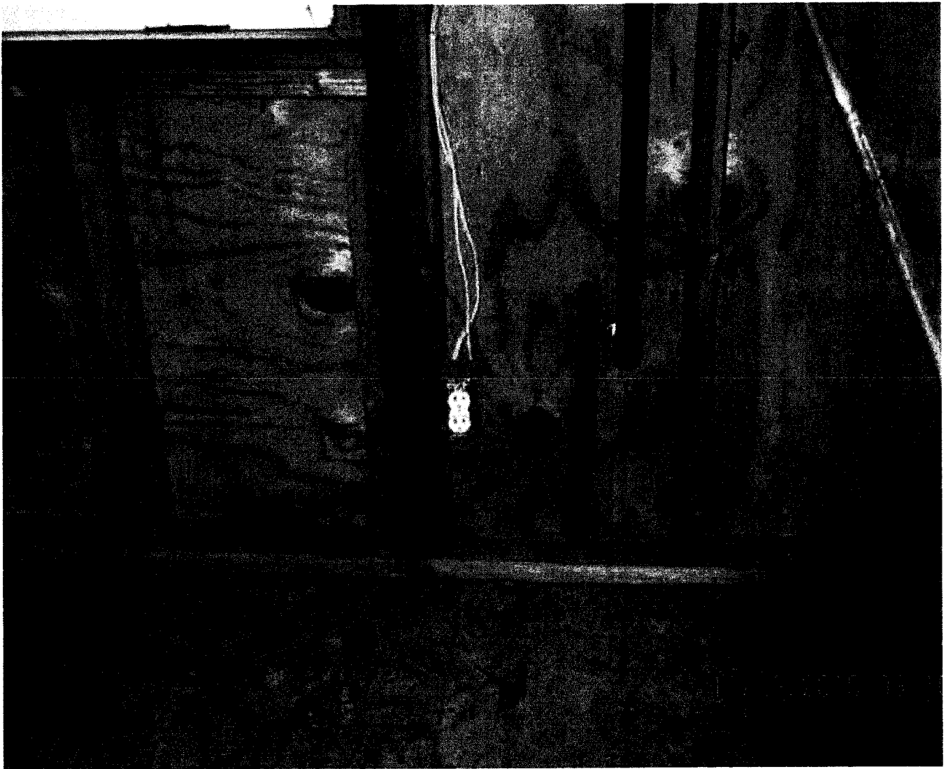
Photo #5 of interior of SSS #1, defects 5,19 no electric; by S. Cervantes - 10/19/2010
