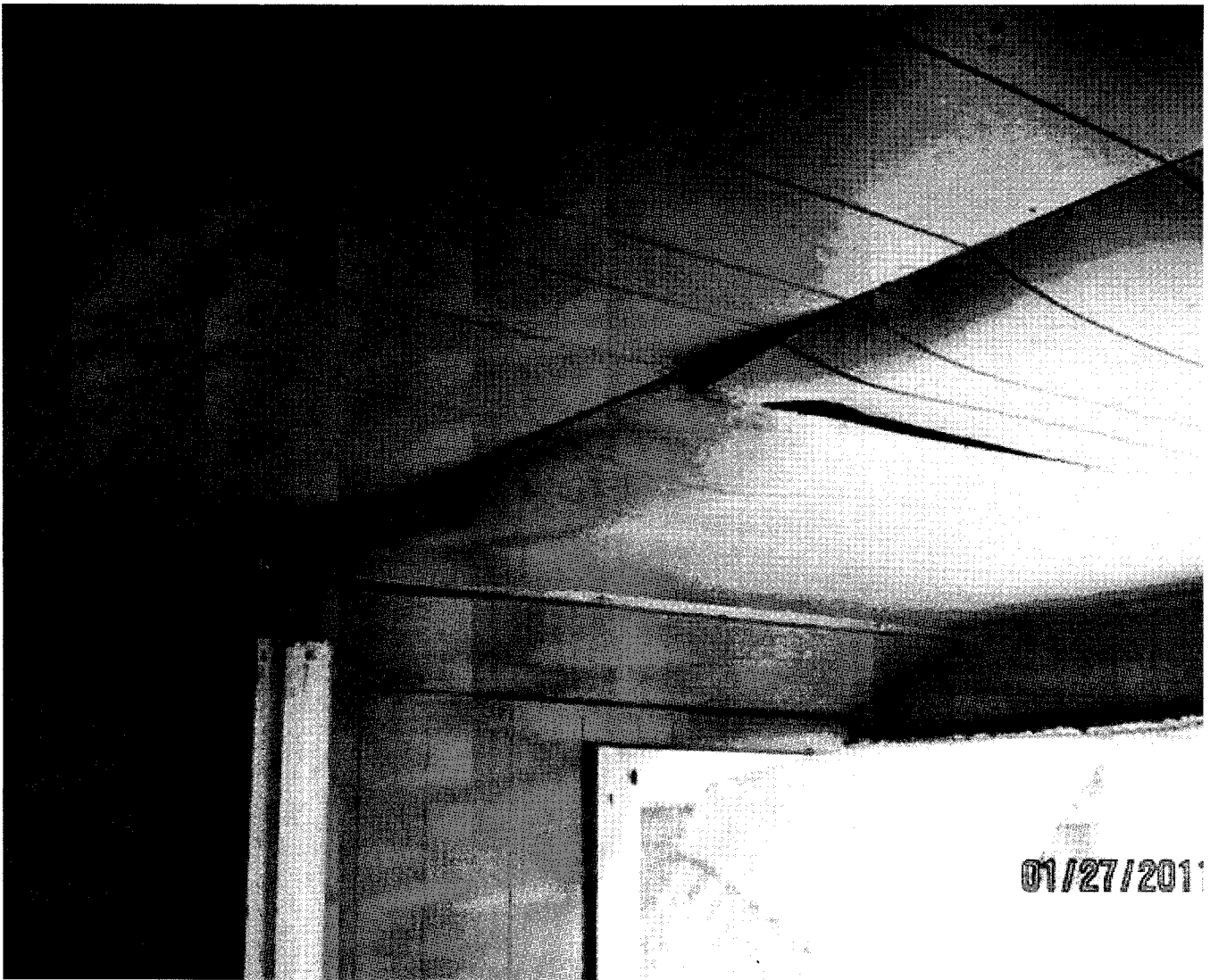
CForrey / SSS#2 - Defect #11, 12 - Leaking roof causing ceiling to detach due to dampness - 01/27/2
