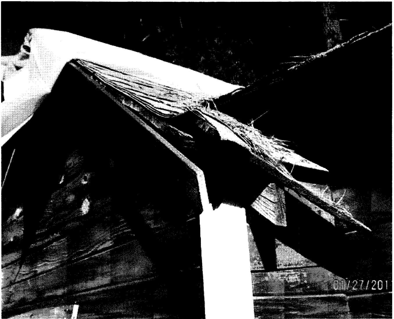
CForrey / SSS #1 Defect #11, roof of small cabin - 01/27/2011
