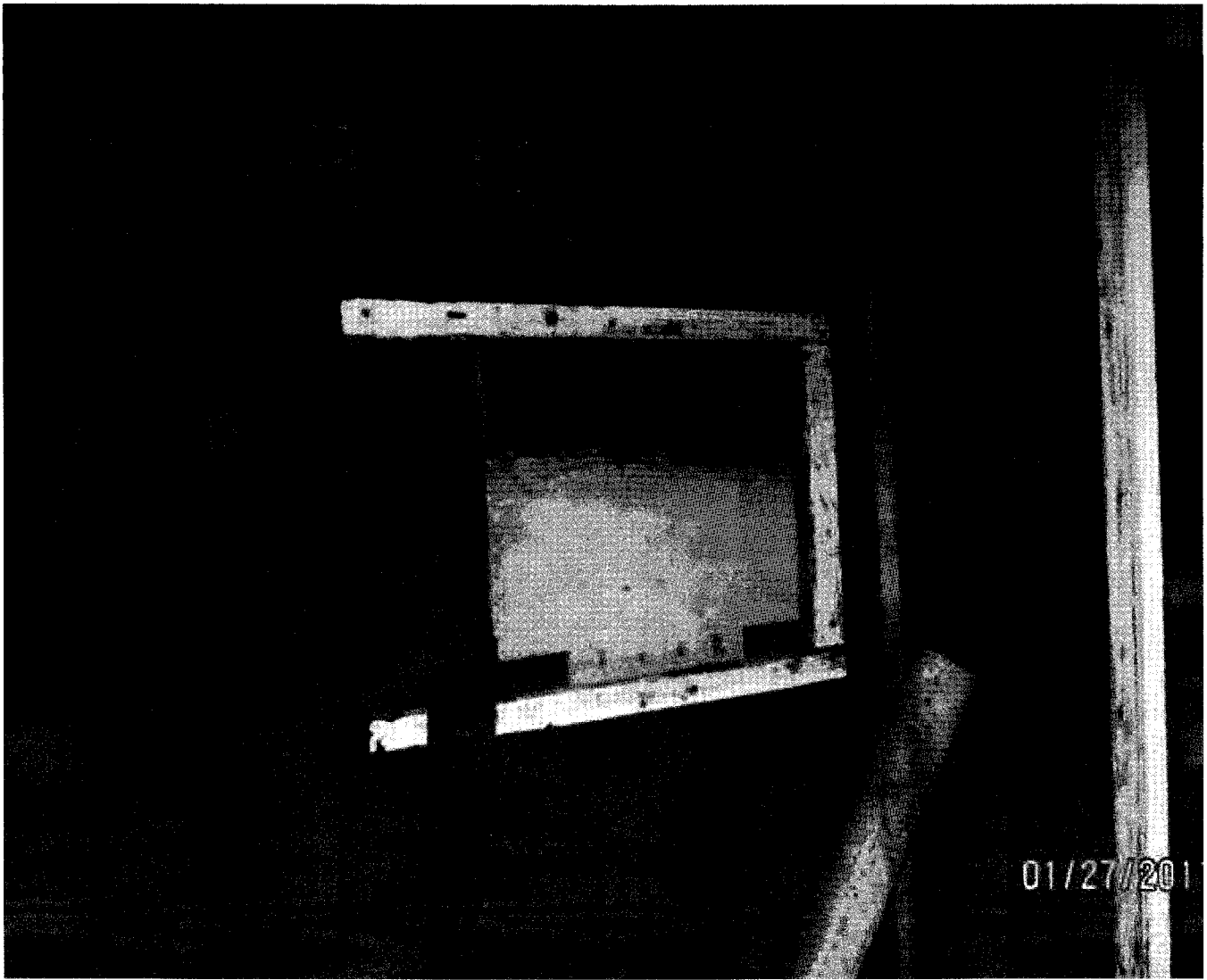
CForrey / SSS#2 - Defects #10, 13, 14 - No protective coating, dilapidation, missing windows - 01/27/
