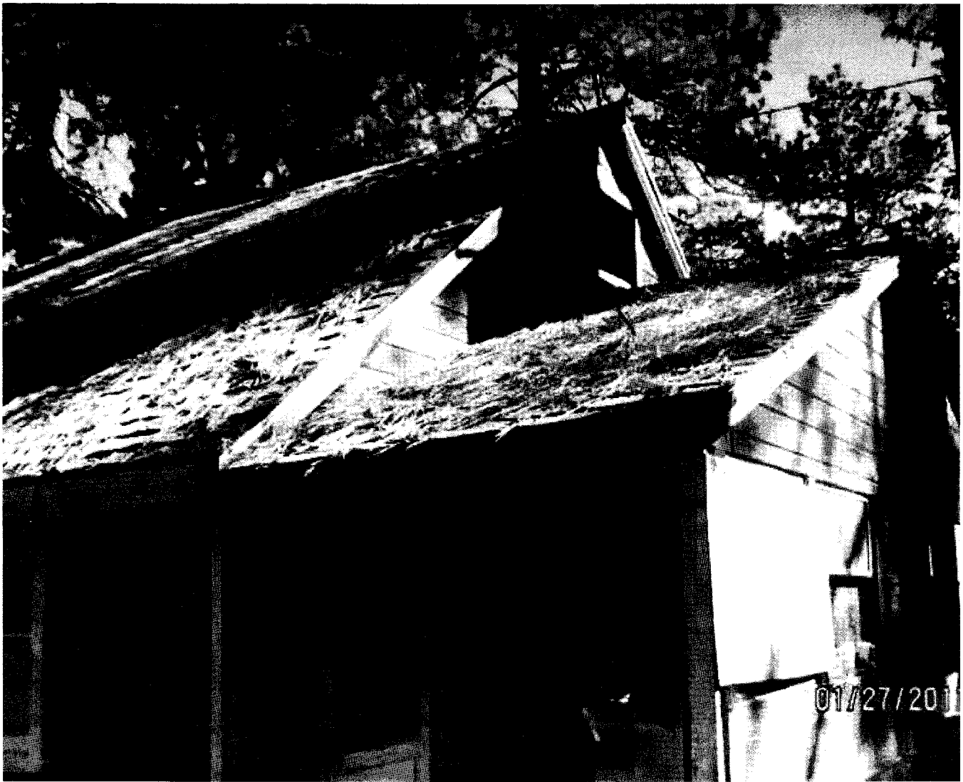
CForrey / SSS #2 - Large Cabin - Defects #10,13,17,14 No protective coating, Missing windows, Aban and accessible to the public, no maintenance - 01/27/2011
