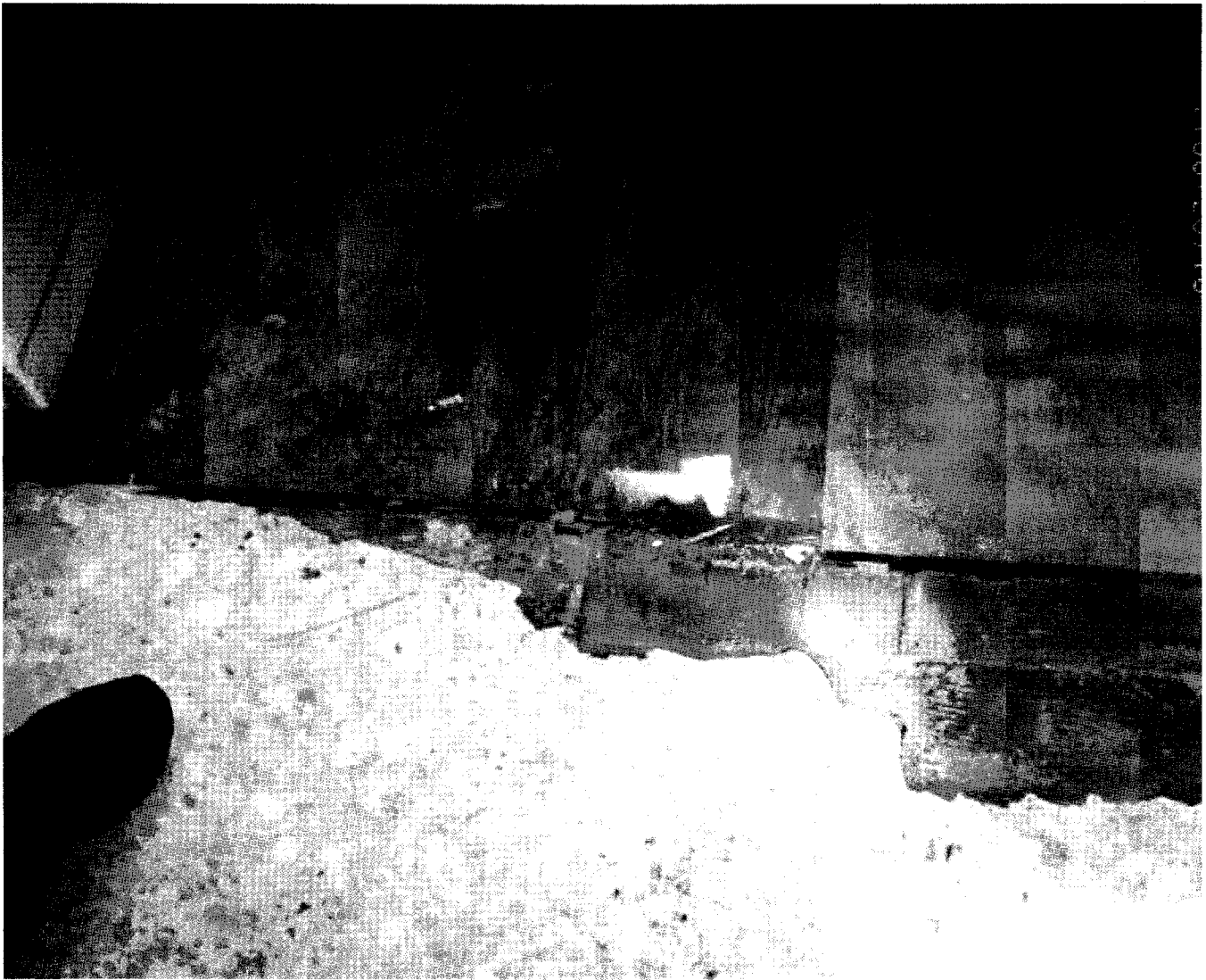
CForrey / SSS#2 - Defect #14 - Flooring dilapidated - 01/27/2011
