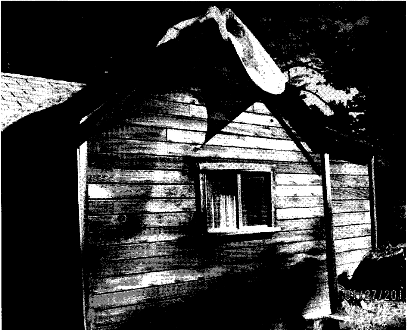
CForrey / SSS #1 - Defect #14, 17- tarp on roof, No protective coating on siding - 01/27/2011
