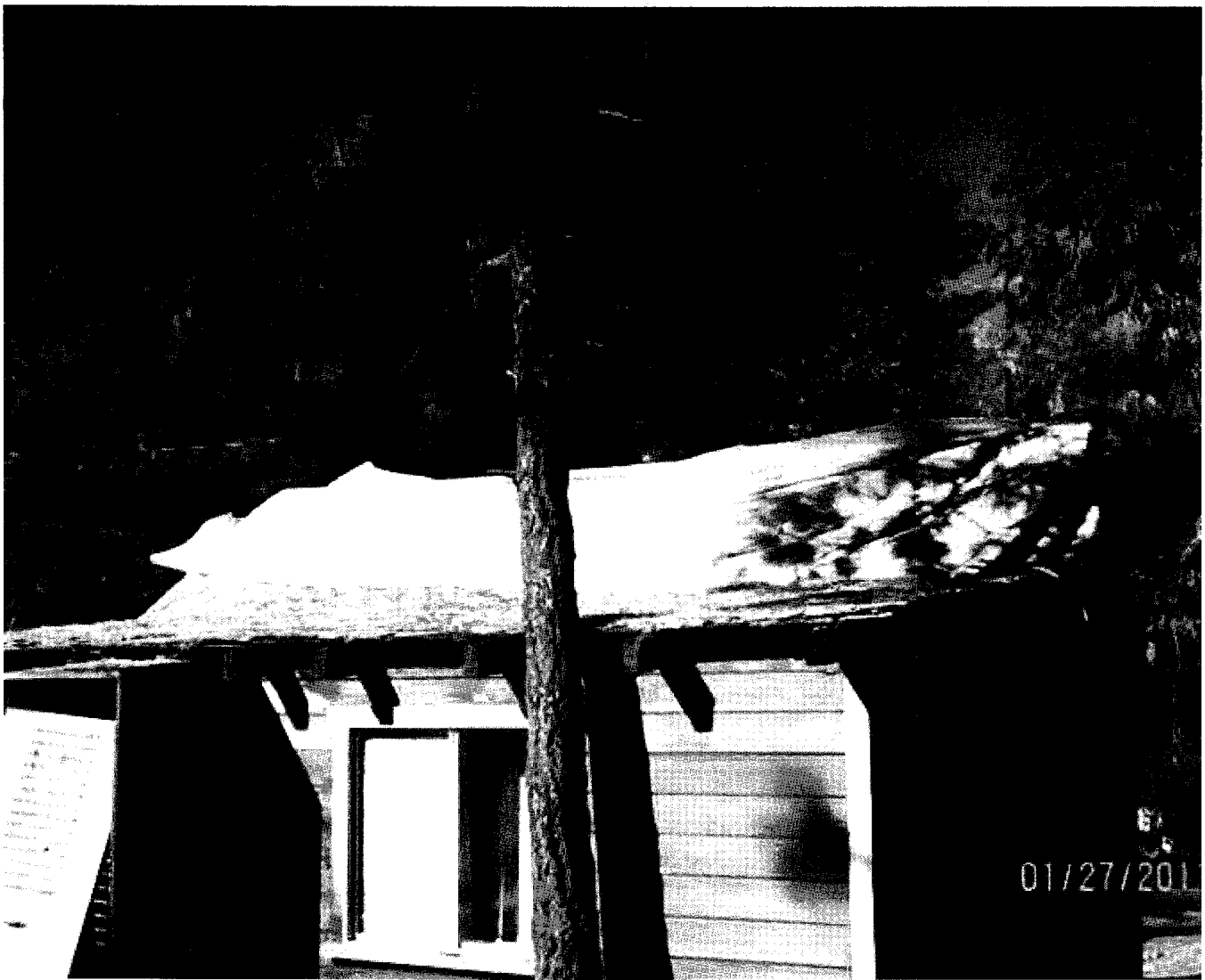
CForrey / SSS #1, Defect # 11 - Tarp as repair for leaking roof - 01/27/2011
