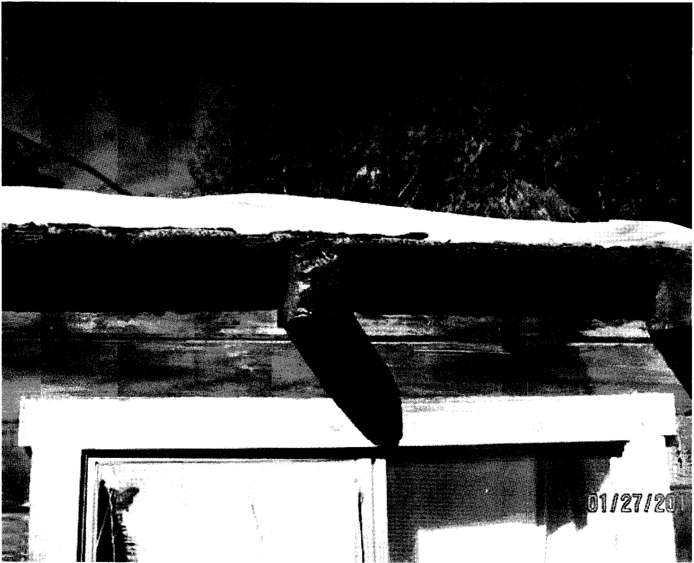
CForrey / SSS #1 Defect #11, 14 - Roof has no maintenance, dilapidation - 01/27/2011
