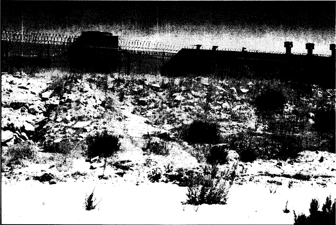
Photo 1A: Portion of Slope to be armored with existing slope armor (courtesy: Tierra Data Inc., 2012).
