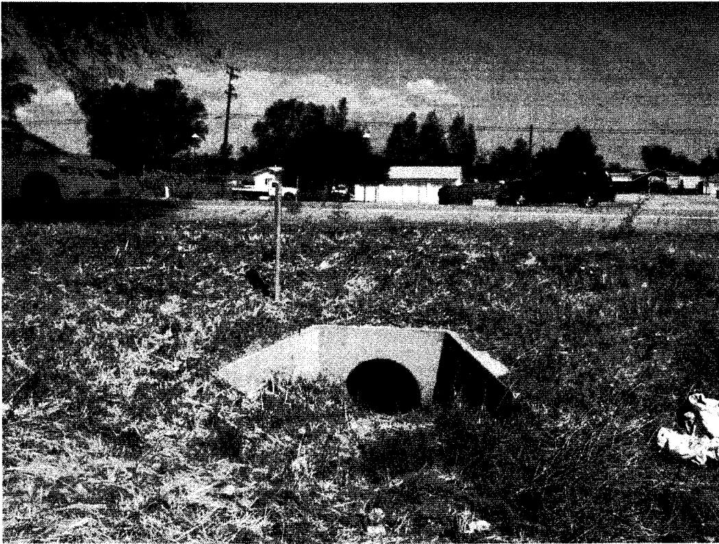
Figure 4 – Photo #1: Outlet of existing facility. Facing east onto Old Highway 215.
