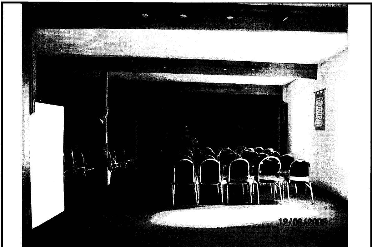
PHOTO # 2 DATE: 12/06/06 TAKEN BY: M. Overholt NOTES: View of sanctuary area at south west portion of church building
