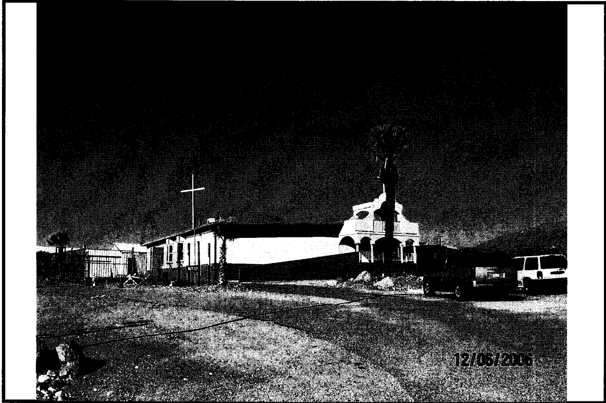
PHOTO # 1 DATE: 12/06/06 TAKEN BY: M. Overholt NOTES: View of building modified/converted to church with façade, handicap ramp & bell tower
