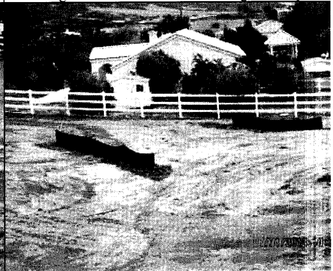
Wagner 80 - Silt fence in segments
