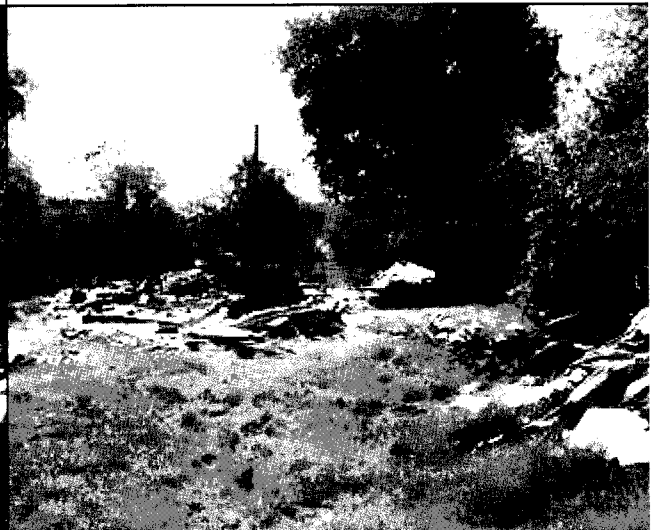
Rubbish (mobile home remains) in the middle of property
