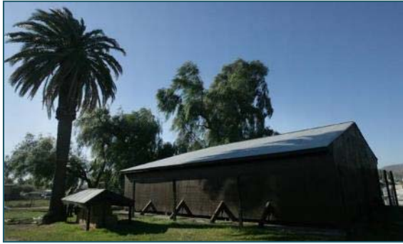
Structure built to preserve the Trujillo Adobe
