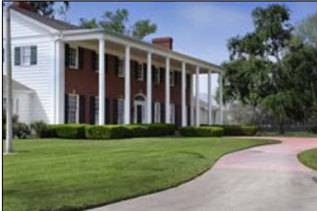
Crestmore Manor Facade
