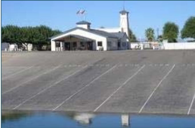
Boat Ramps at Reynolds Resorts
