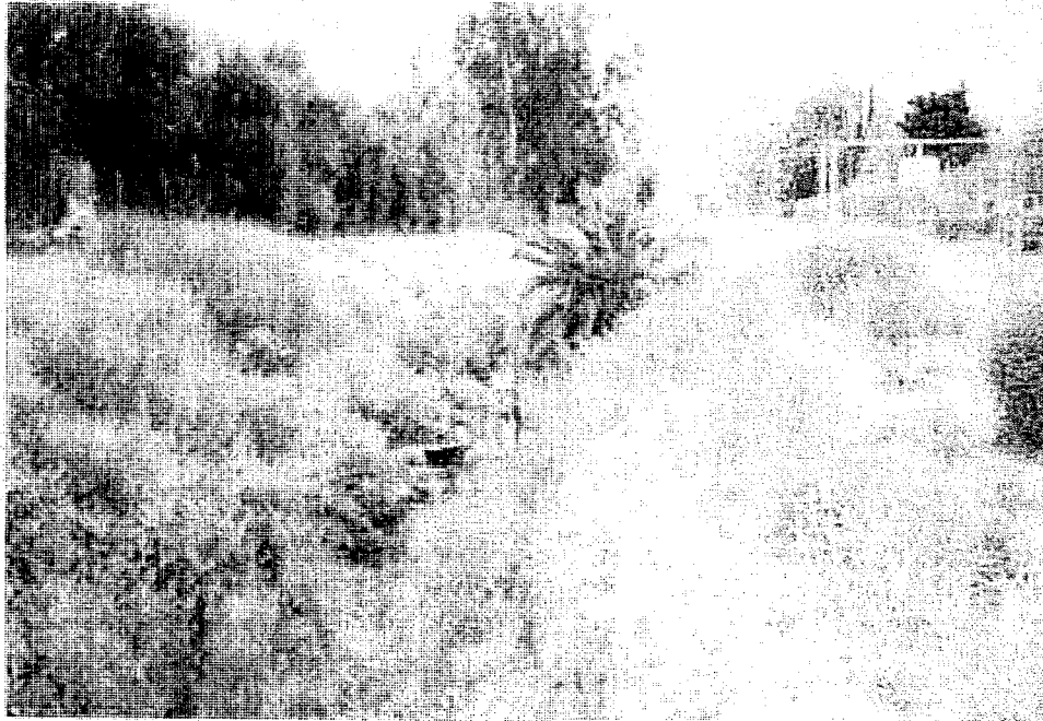
PHOTOGRAPH 3. This photograph depicts the North Norco Flood Control Channel on the east end of the channel as it transitions into the improved concrete channel. Photograph taken looking east on 9-11-2008.
