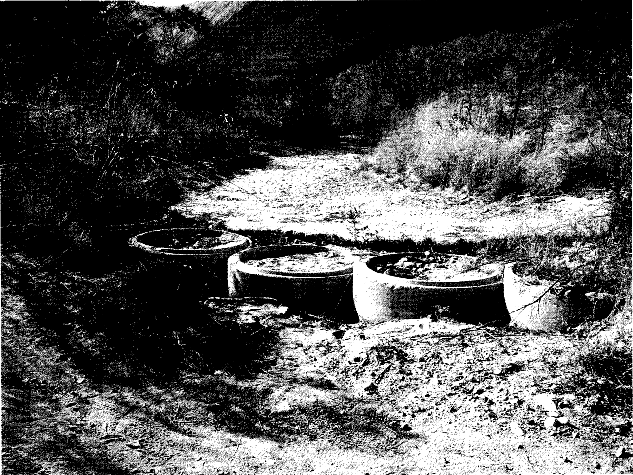
Figure 3A – Westerly view of Aliso Canyon crossing. Access road is in the forefront.
