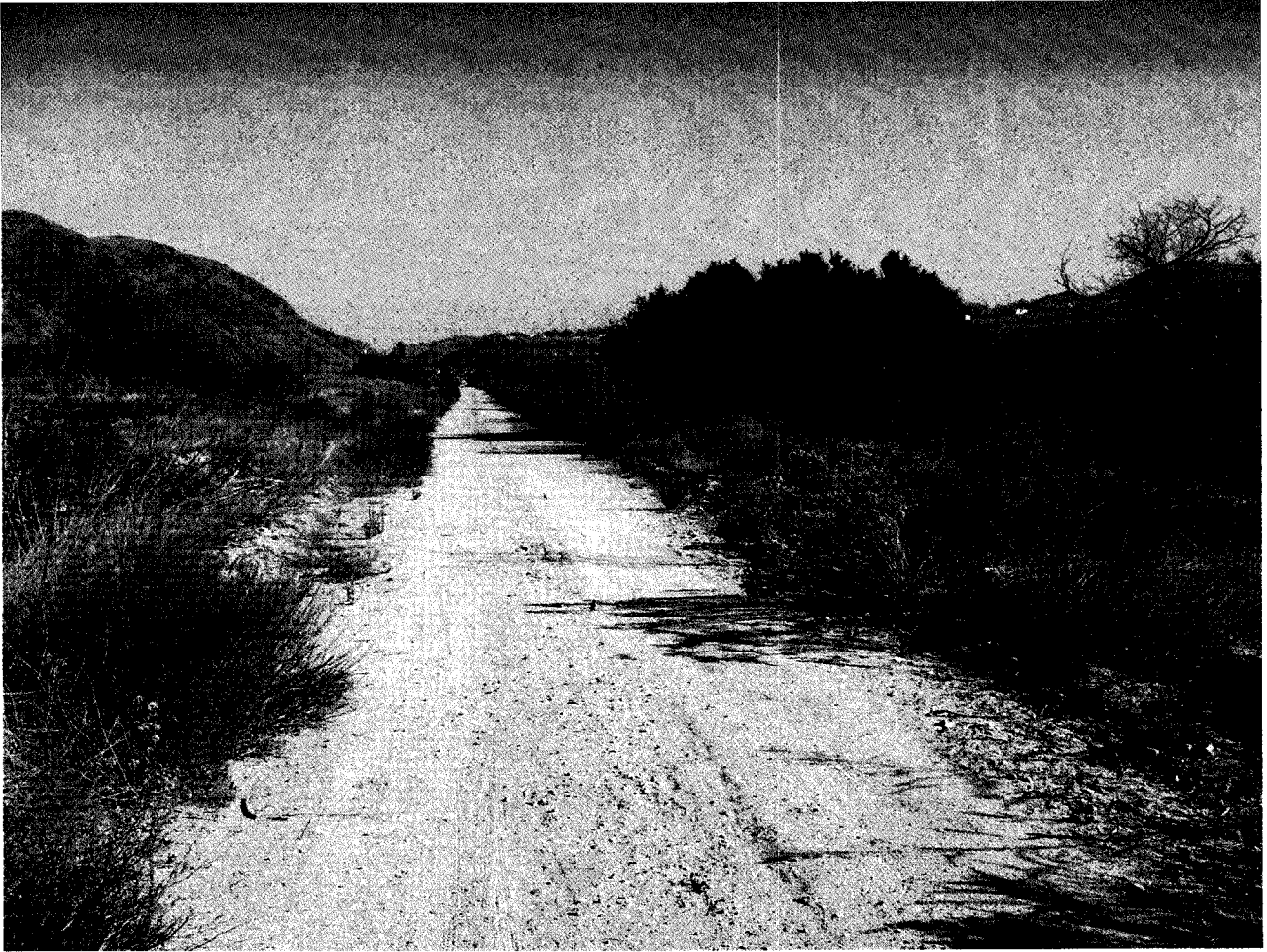
Figure 3B – Easterly view of Project site along the Brine Line Maintenance Road.
