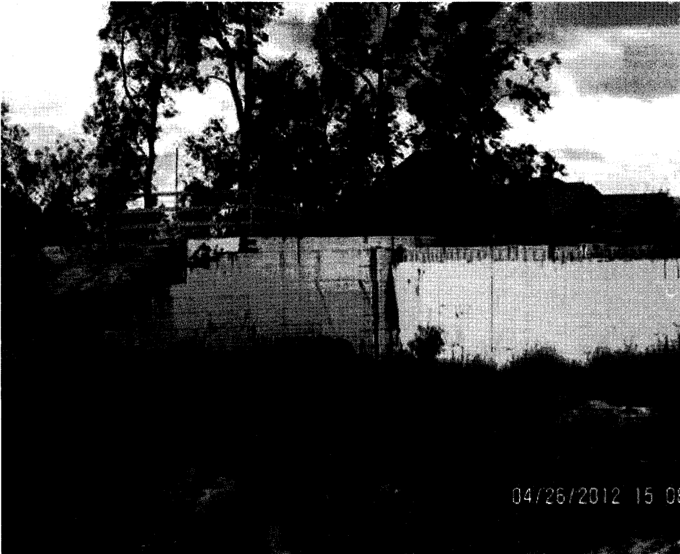
Wagner 80 - Retaining wall / pool. - 04/26/2012
