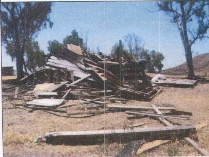
05/01/13 - Pile of burnt rubbish, taken from north end facing south. L Lyon
