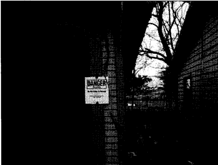
Posted Danger Do Not Enter Sign on Structure #1
