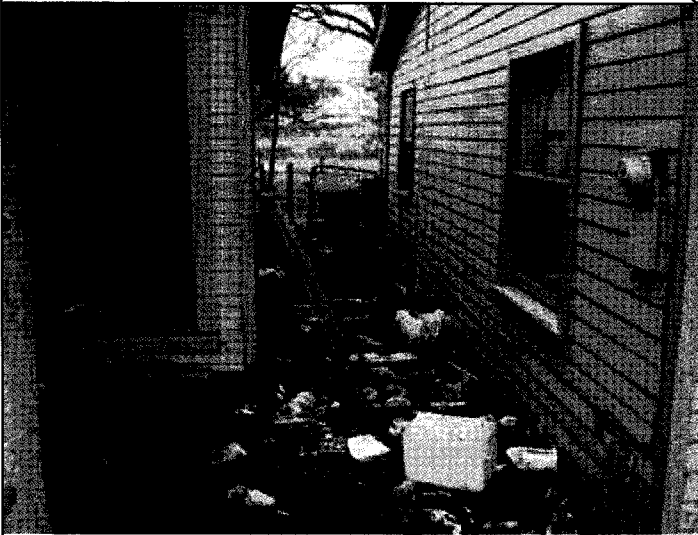
Rubbish between the two structures
