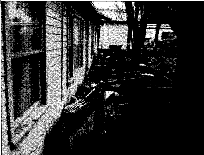
Front of Building #2
