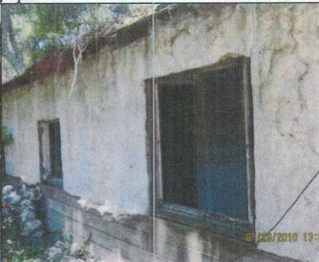
J.Wagner #80 Windows missing. Faulty weather protection
