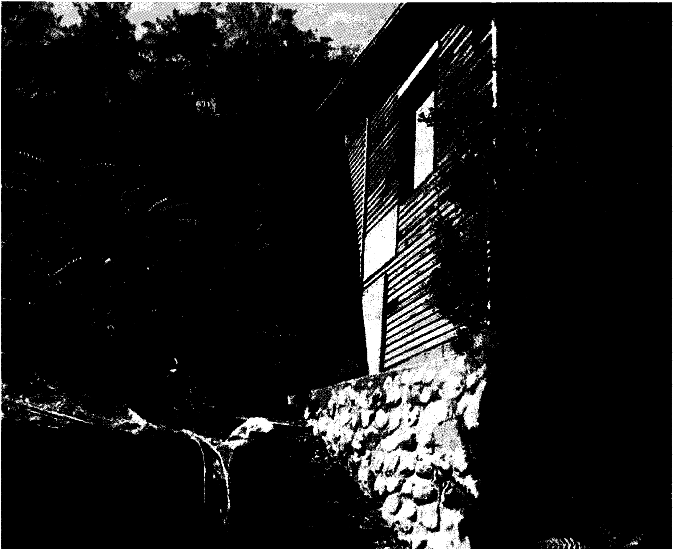
Structure #2- Red house. J. Palmer - 09/26/2012
