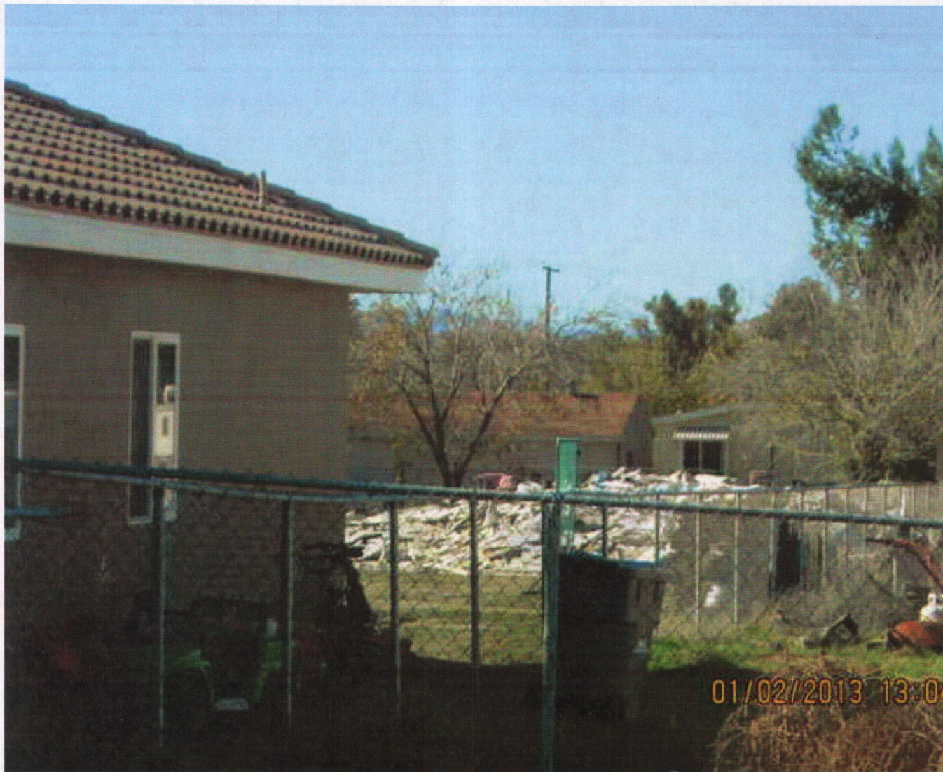
Demo Drywall at rear of property. Lpadilla - 01/02/2013
