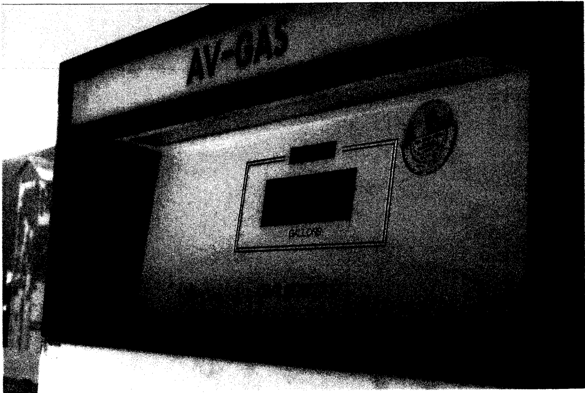
BLYTHE AIRPORT – 2006 WEIGHTS AND MEASURES CERTIFICATION SEAL – DAMAGED, SHOWING ONLY HALF OF SEAL ON FRONT OF FUEL PUMP ATTACHMENT "B"
