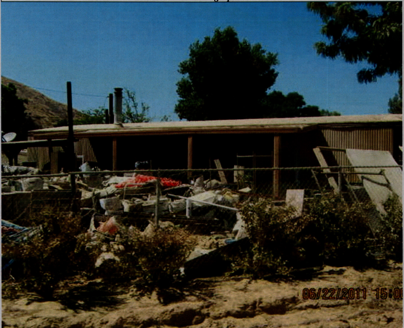
Excessive Outside Storage - Pike - 06/22/2011
