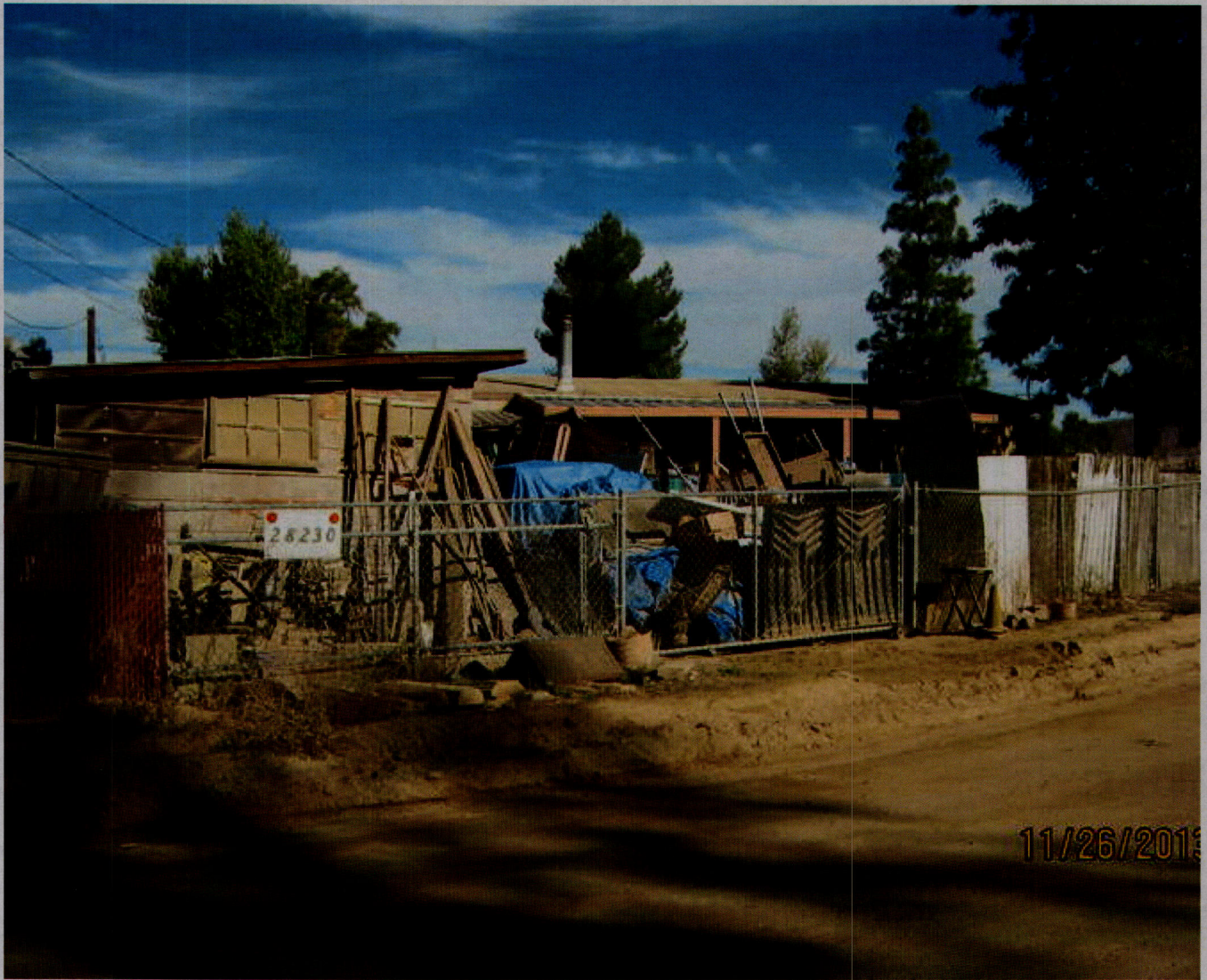
excessive outdoor storage and rubbish - 11/26/2013
