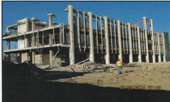
Figure 3. July 22, 2014: Demolition of Third Floor, CAC Building, Southwest View
