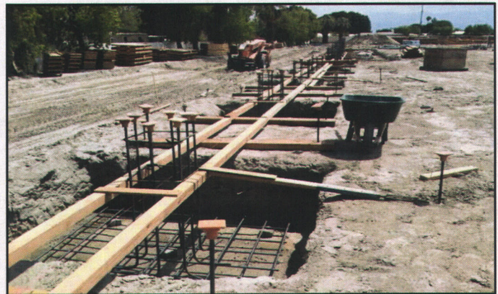
Figure 10. August 01, 2014: Spread Footings with Column Reinforcement
