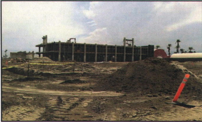
Figure 7. August 01, 2014: Southwest View, Late July
