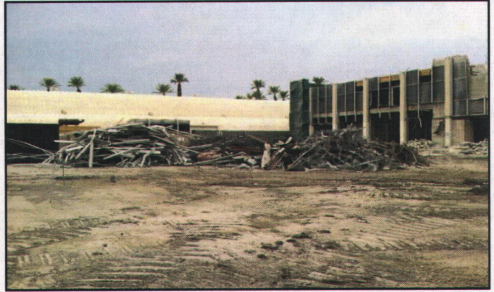
Figure 8. August 01, 2014: Steel and Metal Demolition Debris
