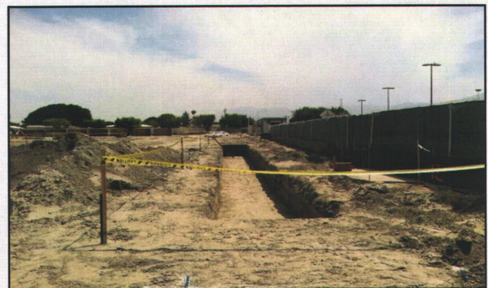
Figure 6. August 01, 2014: Grade Beam Foundation
