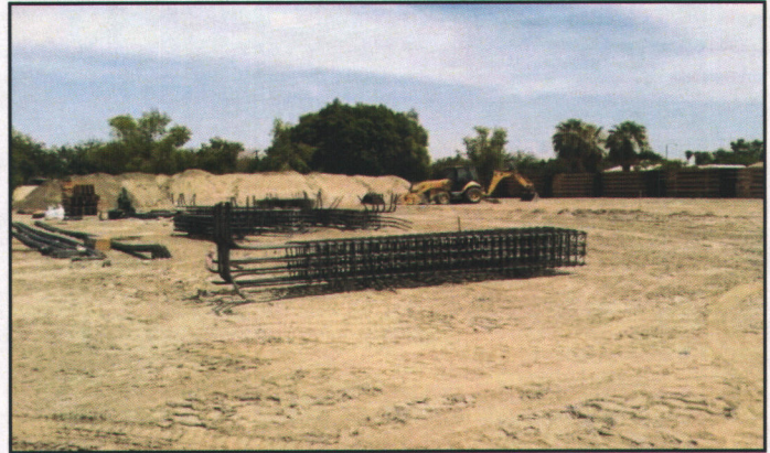
Figure 8. August 01, 2014: Ground Level Steel Reinforcement
