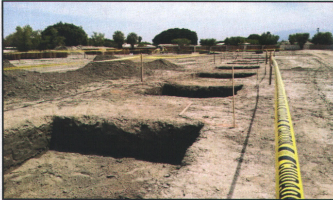
Figure 7. August 01, 2014: Spread Footing Foundation
