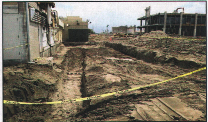
Figure 10. August 01, 2014: Grease Interceptor Trenching for Replacement at Existing Jail
