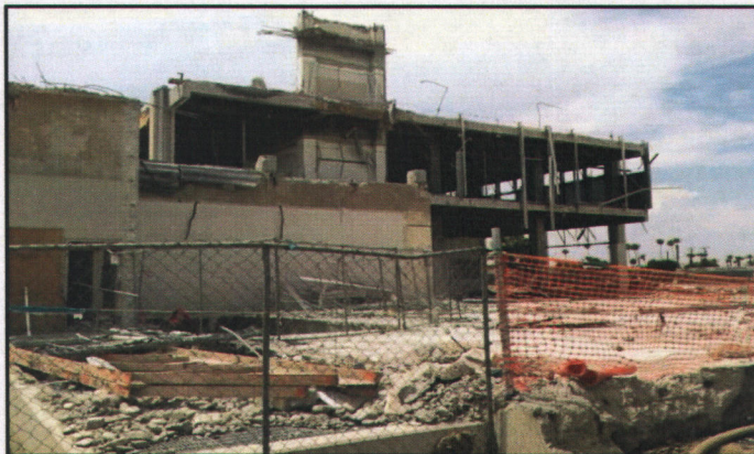
Figure 9. August 01, 2014: CAC Building, Roof, Fourth and Third Floor Removed
