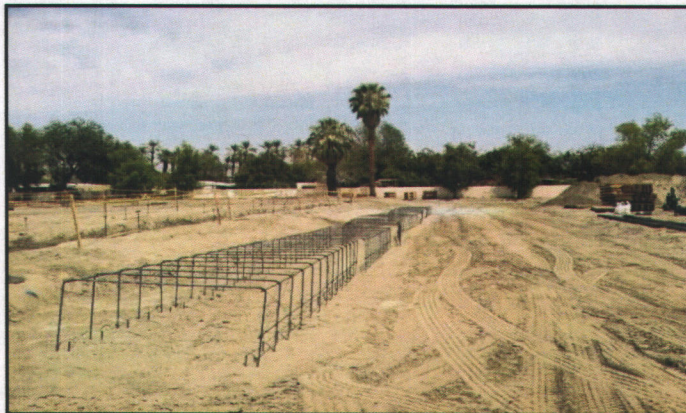
Figure 9. August 01, 2014: Foundation (Grade Beam) Steel Reinforcement
