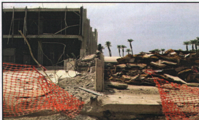
Figure 11. August 01, 2014: View North at CAC Building Demolition
