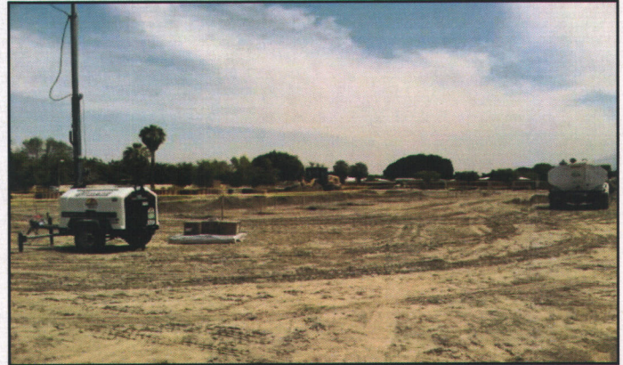
Figure 2. August 01, 2014: South East View
