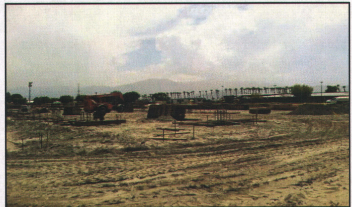
Figure 4. August 01, 2014: Southwest View
