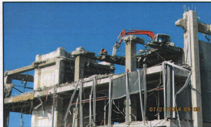
Figure 5. July 21, 2014: Demolition Crew and Equipment at Third Floor
