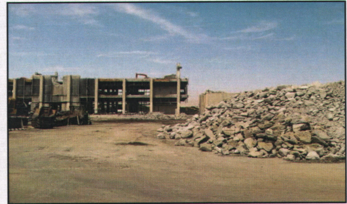
Figure 6. August 01, 2014: North View, Late July
