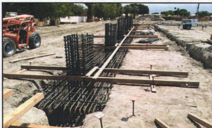
Figure 11. August 01, 2014: Reinforced Grade Beam with Column Reinforcement
